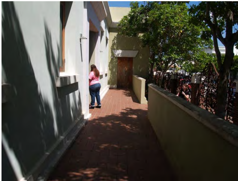
Figure 3. Elevated platform that provides access to the three entrances on the main façade. In the 2002 rehabilitation, as it was originally build, wooden doors where installed once again.
