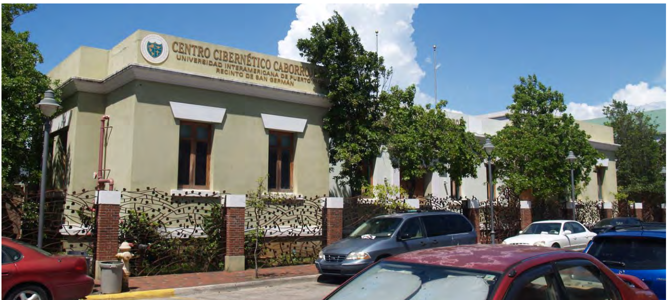
Fig. 2. Main façade. Central volume recedes back, while the flanking volumes project outward.
