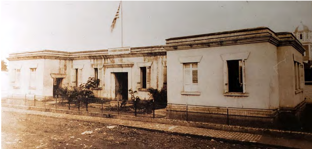
Figure 13. The James L. M. Curry Graded School , ca. 1910. (Colección A. Moscioni, Colección Puertorriqueña, Universidad de Puerto Rico, Recinto de Rio Piedras). Moscioni's photo shows distinguishable features still found in today's building: same footprint, openings, moldings, etc. It also shows that the sidewalk directly in front of the school received a special treatment in its texture to emphasize the school's special location and significance. Currently, the 21st century fence and sidewalk in front of the building resemble a similar treatment.
