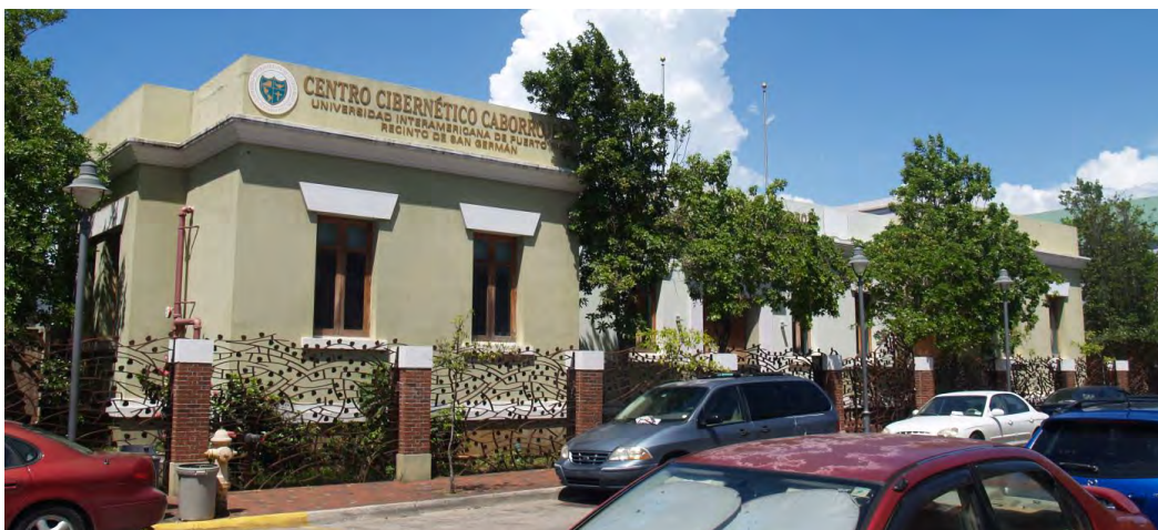
Figure 15. The James L. M. Curry Graded School Building, 1903/2019.
