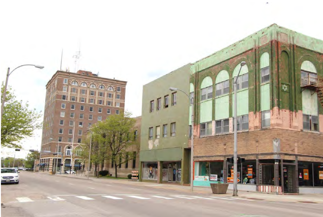
Photo 14. The south side of 200 block of W. 2 nd Street, view facing southeast.
