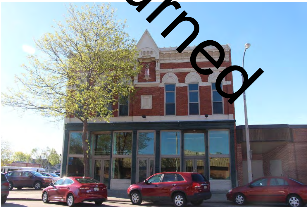
Photo 2. The Grand Army of the Republic (GAR) Building (HL06-135, 1886), 215 E. 3 rd Street, view facing southwest.
