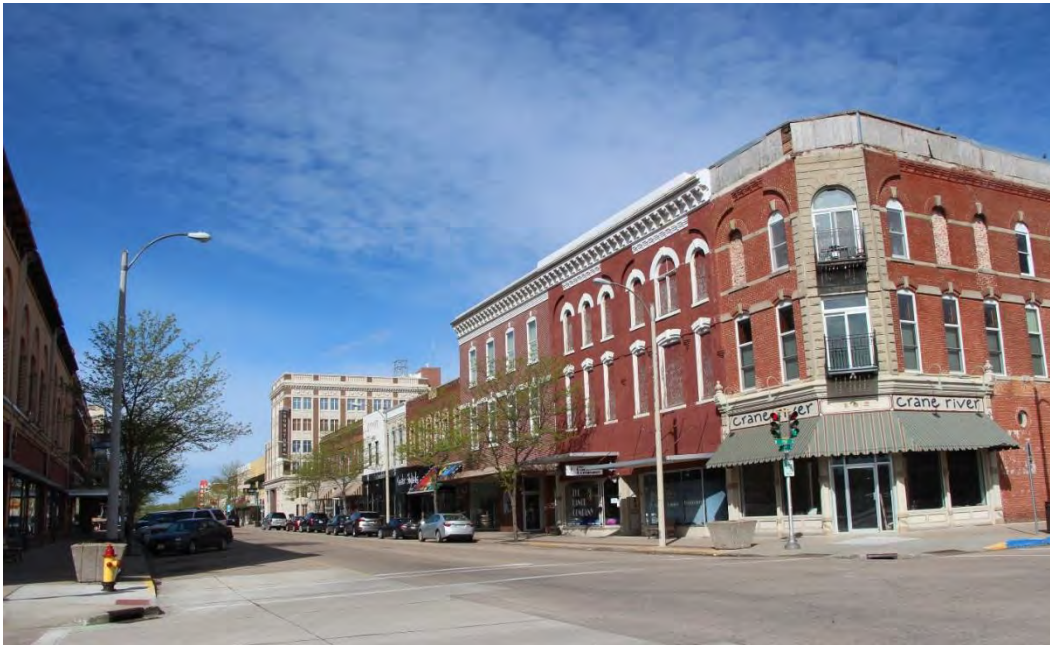
Photo 5. The north side of the 100 block of W. 3 rd Street, view facing northwest.
