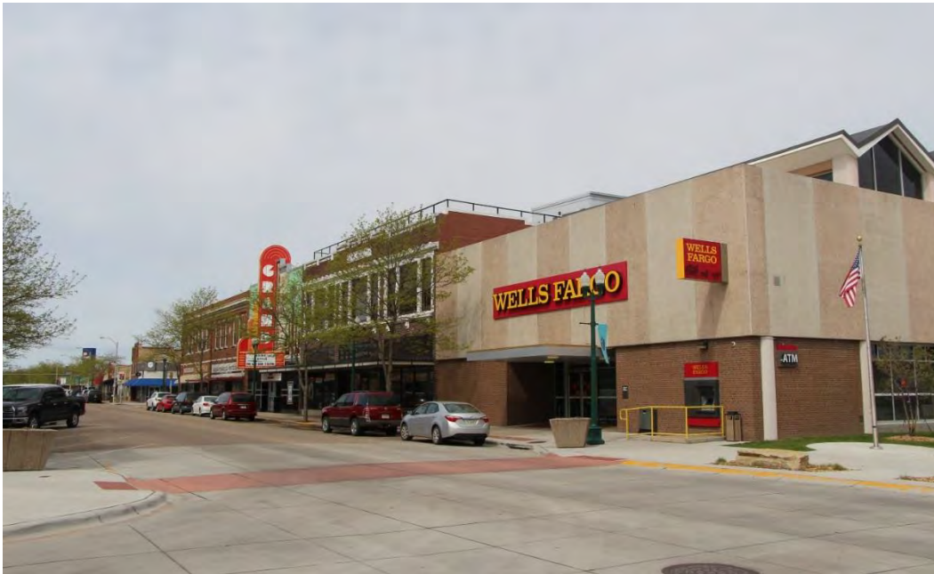
Photo 9. The north side of the 300 block of W. 3 rd Street, view facing northwest.
