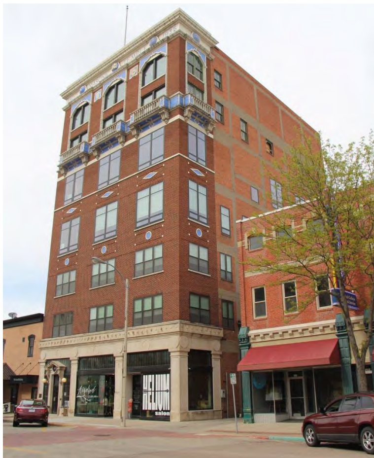
Photo 20. The Masonic Building (HL06-017), 217 N. Locust Street, view facing northeast.
