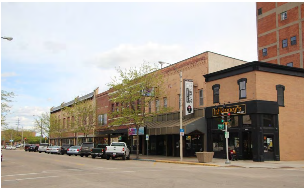
Photo 6. The south side of the 100 block of W. 3 rd Street, view facing southeast.
