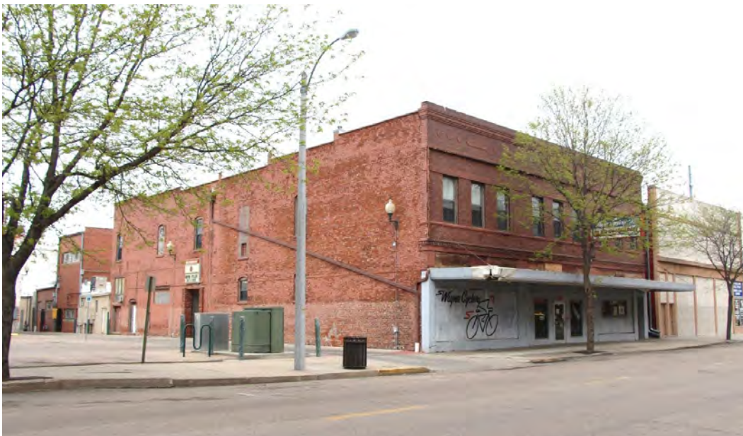
Photo 18. The east side of 300 block of N. Pine Street, view facing southeast.
