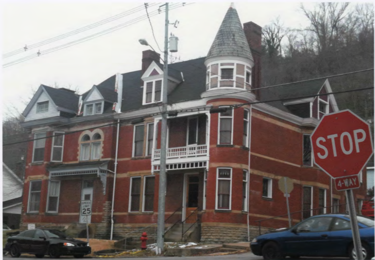
KY_MASON CO_COX BLDG_0011
