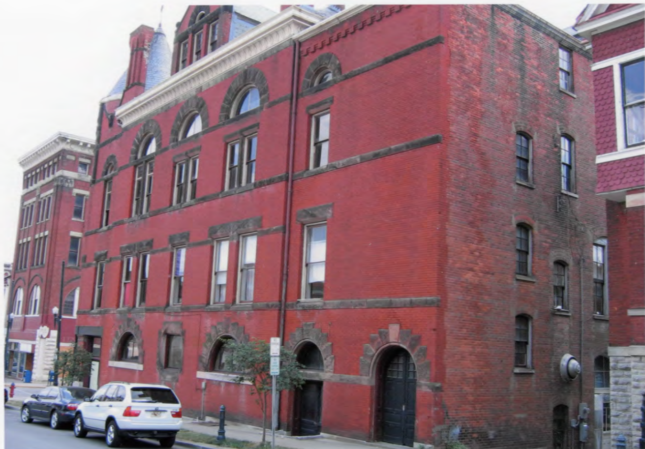
KY_MASON CO_COX BLDG_0003
