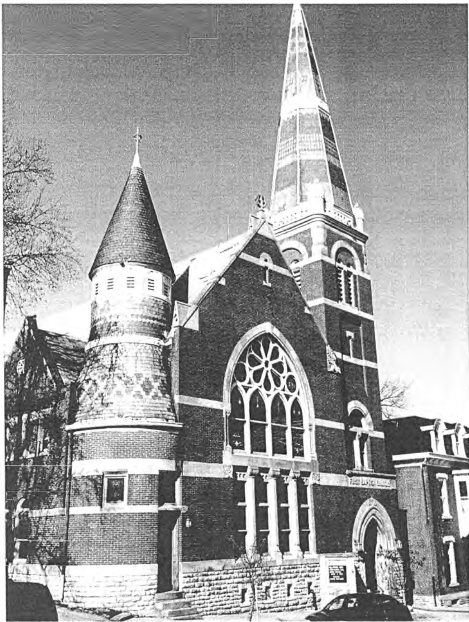
Photo 13 (Above). First Baptist Church. MS-M-132. Mason County, Ky. Market Street Facade. Looking NW
