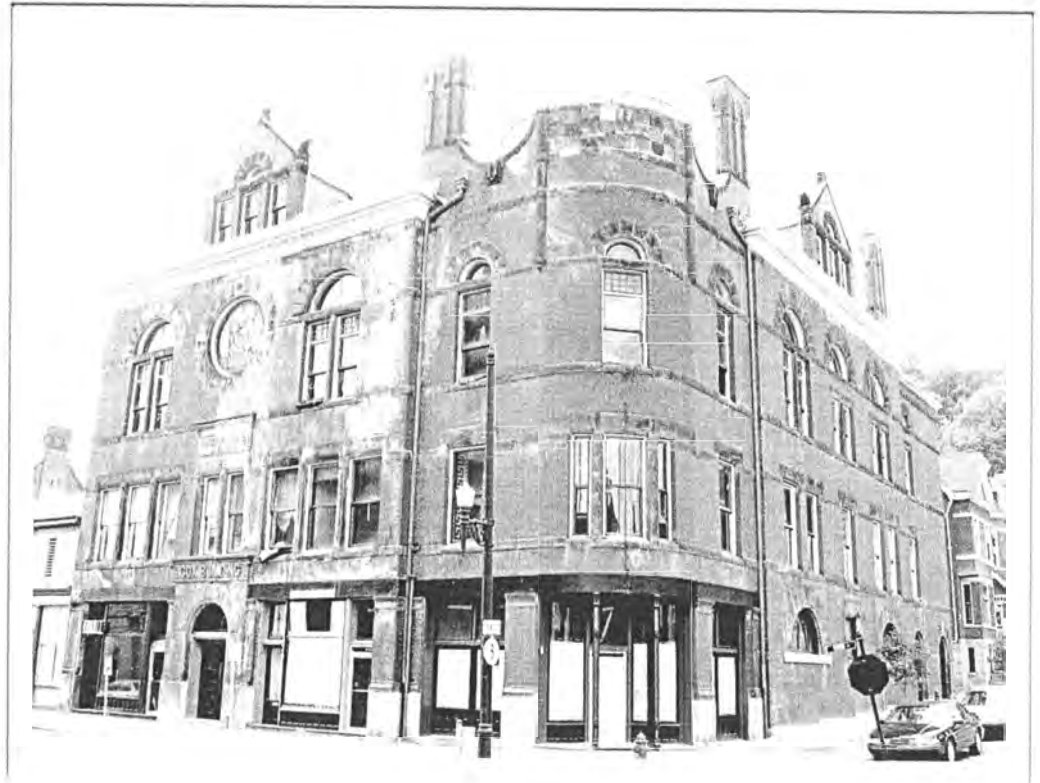
Photo 2 (Left) The Cox Building, MS-M-III, Mason County, Ky. North (3rd St) Facade, Looking SSE Orloff Miller, 2007, author's collection.
