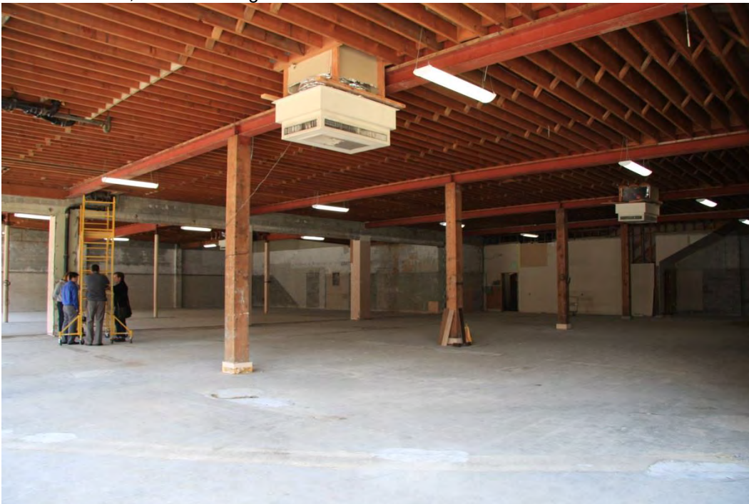
Photo #9 of 15 (WA_PierceCounty_RentonWoolworthBld_0009) Main floor interior I, west (left) and north (right) elevations, camera facing northwest
