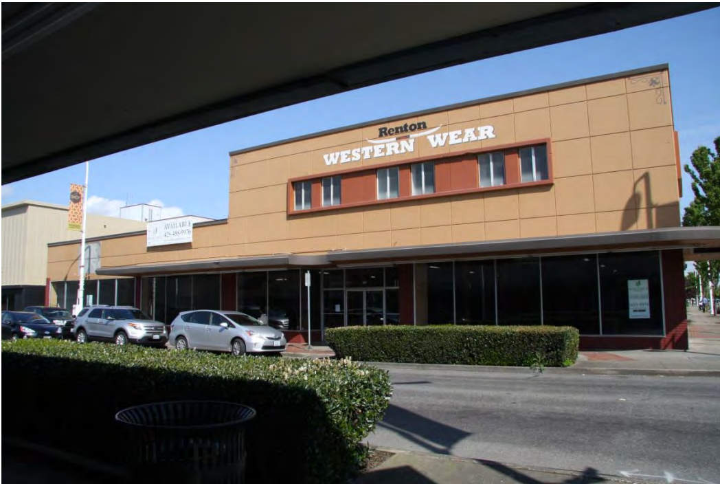
Photo #2 of 15 (WA_PierceCounty_RentonWoolworthBld_0002) South façade, camera facing northwest
