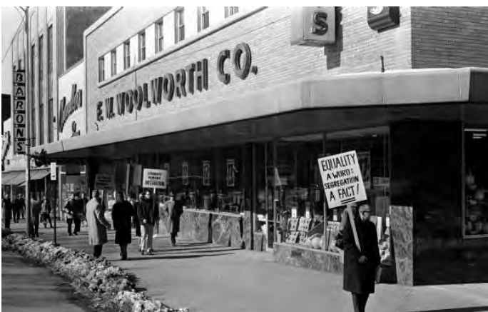
Madison, WI – Woolworth Co. Store (built 1954)
