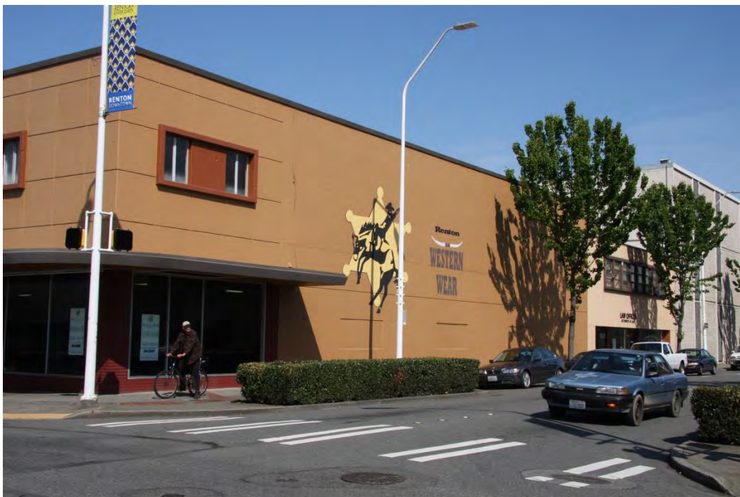
Photo #5 of 15 (WA_PierceCounty_RentonWoolworthBld_0005) East elevation, camera facing northwest
