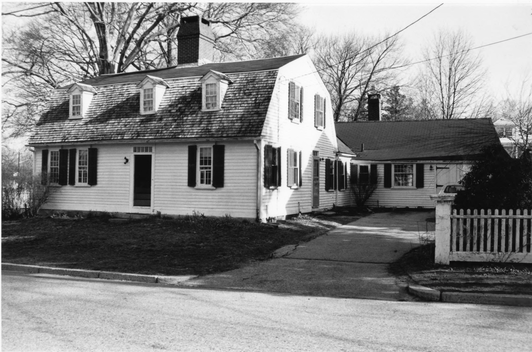
Whipple-Angell-Bennett House Providence County, R.I. Photo # 2 of 8
