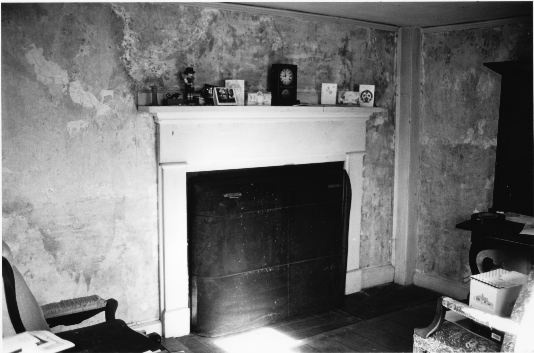
Whipple-Angell-Bennett House Providence County, R.I. Photo #6 of 8
