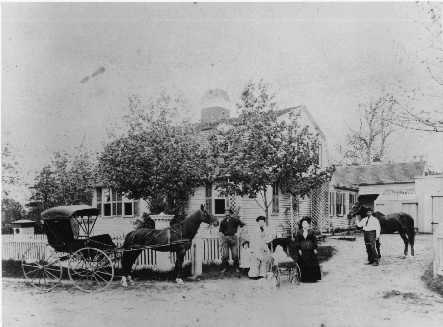
Whipple-Angell-Bennett House Providence County, R.I. Photo # 1 of 8
