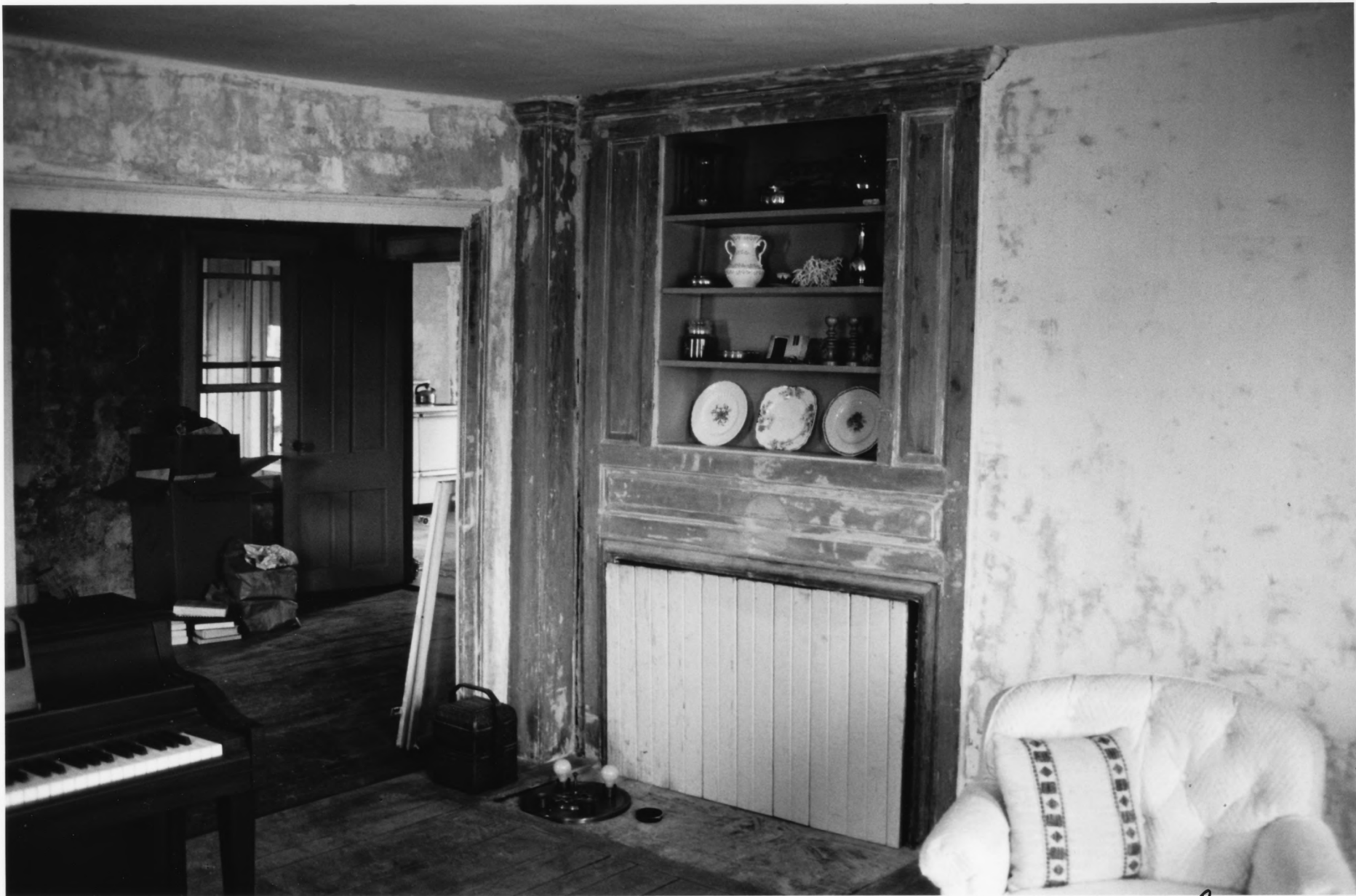
Whipple-Angell. Bennett House Providence County, R. I. Photo # 5 of 8
