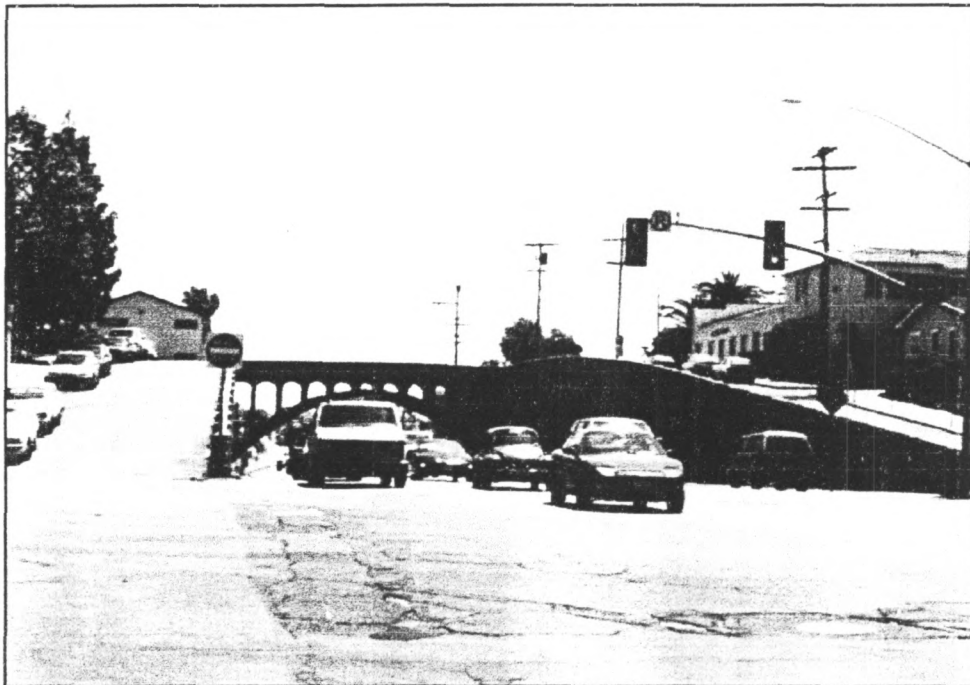
Photograph #1 Georgia Street Bridge/University Avenue Grade Separation Cut Retaining Walls San Diego County, CA Photograph Taken by Alex D. Bevil May 1998 Original Negative in Possession of Photographer View of Western Approach to Grade Separation Cut, Looking East along University Avenue from Intersection of University Avenue and Park Boulevard
