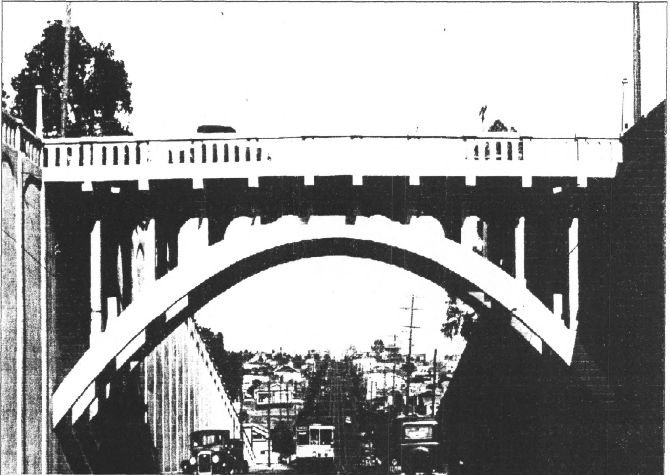
Georgia Street Bridge and University Avenue Grade Separation Cut Retaining Walls San Diego County, CA San Diego Historical Society—Photograph Collection Close-up of Photograph #6852 Showing Bridge Detail and Approaching Electric Streetcar Under Arches
