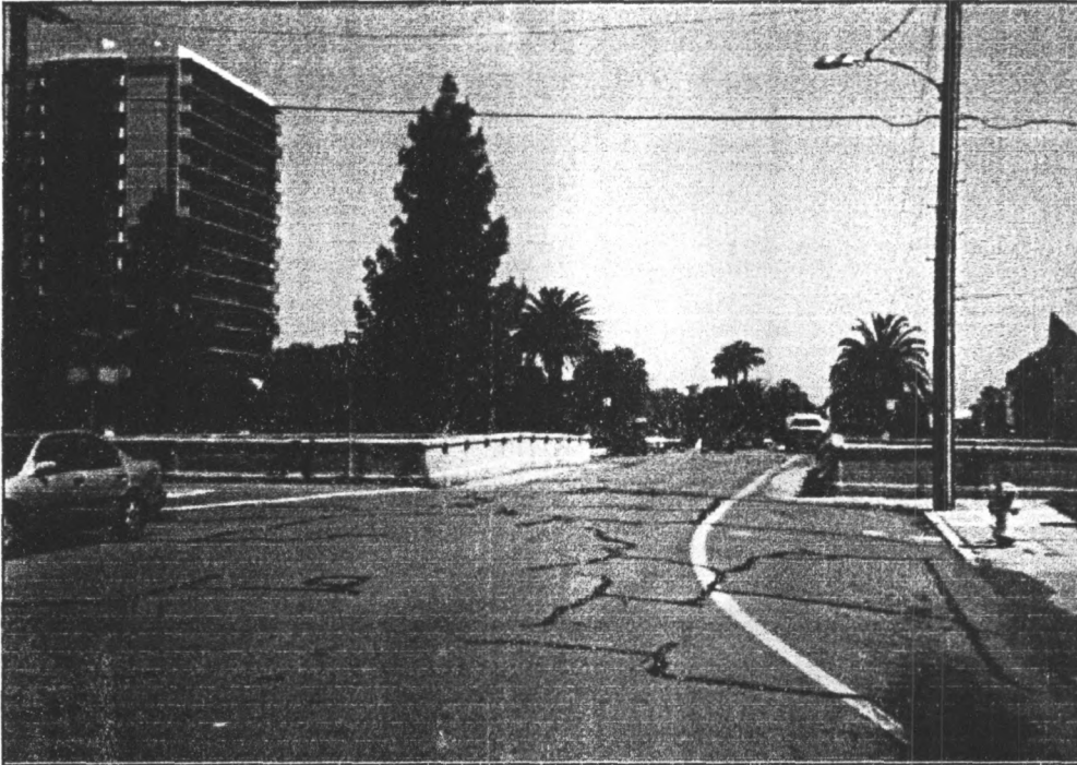
Photograph #3 Georgia Street Bridge/University Avenue Grade Separation Cut Retaining Walls San Diego County, CA Photograph Taken by Alex D. Bevil May 1998 Original Negative in Possession of Photographer View of Southern Approach to Bridge Deck, Looking North along Georgia Street toward University Heights
