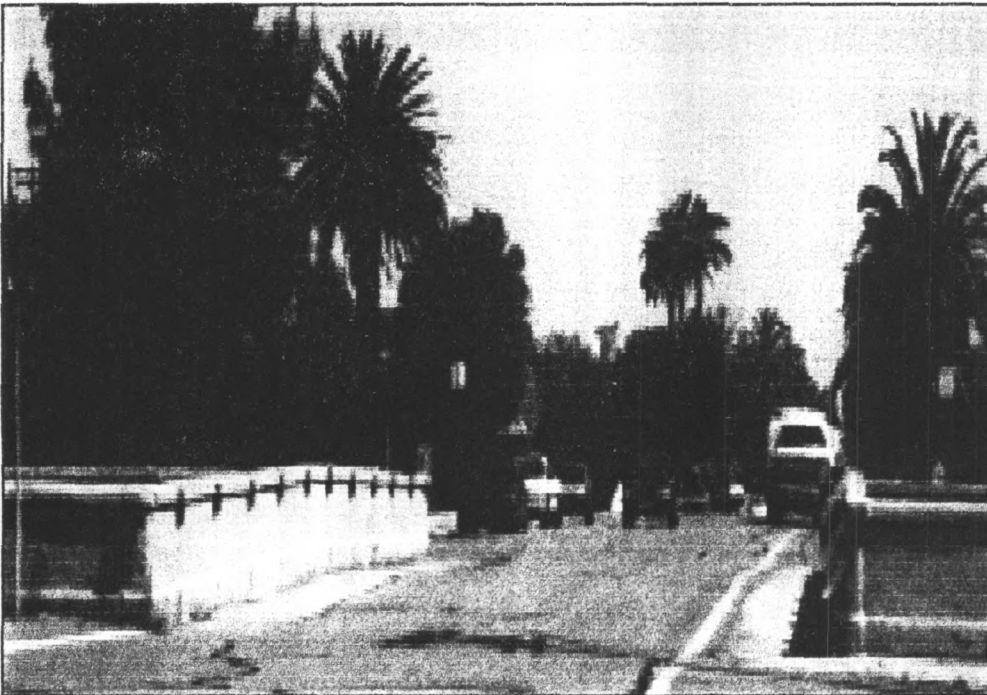
Photograph #3a Georgia Street Bridge/ University Avenue Grade Separation Cut Retaining Walls San Diego County, CA Photograph Taken by Alex D. Bevil May 1998 Original Negative in Possession of Photographer View of Southern Approach to Bridge Deck, Looking North along Georgia Street toward University Heights Close-up Detail of Sidewalk along Roadbed
