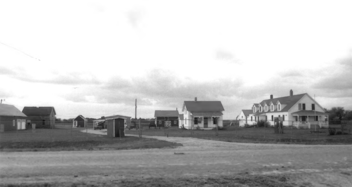
BAGG BONANZA FARM Richland County, North Dakota Panorama of buildings west of County Road Photo by J. Caywood, 10/01
