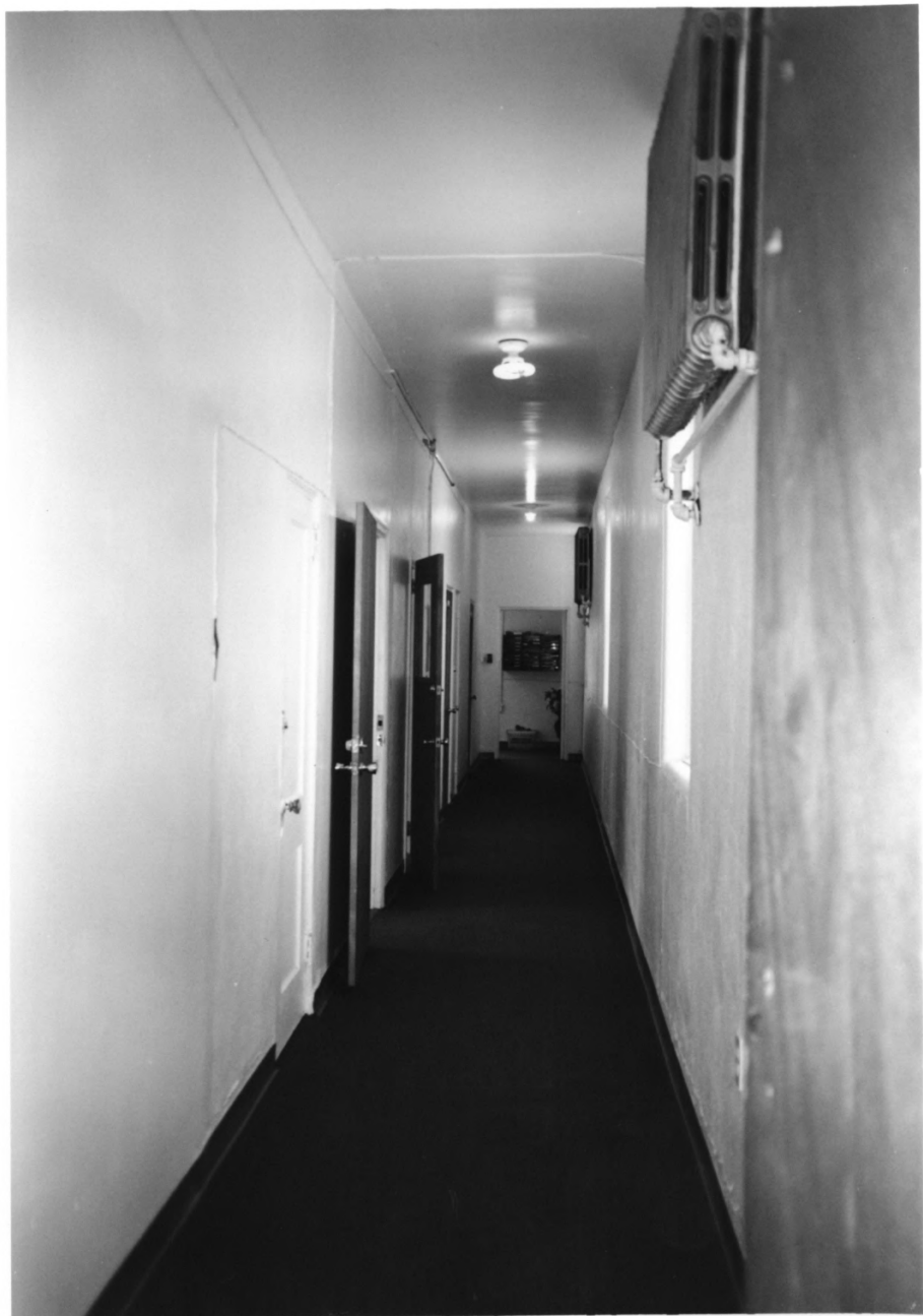
PHOTO 9 OF 13. COMMUNITY HOSPITAL. NEWARK, ESSEX CTY. NJ
