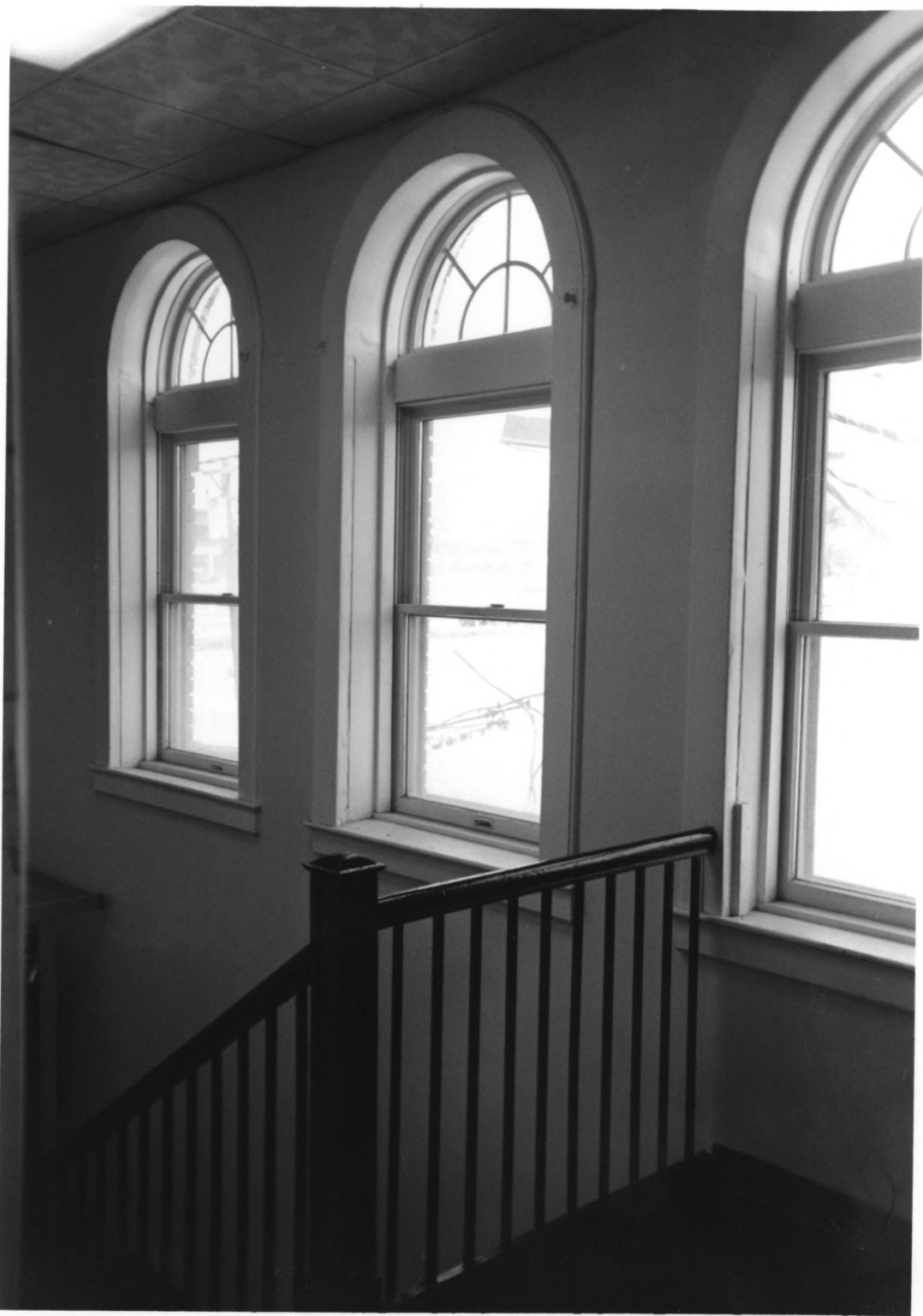
PHOTO 8 OF 13. COMMUNITY HOSPITAL. NEWARK, ESSEX CTY. NJ
