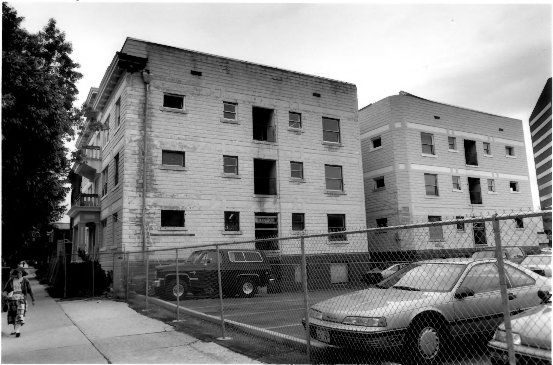
HOLLYWOOD APARTMENTS SALT LAKE CITY, SALT LAKE CO., UTAH PHOTO #2
