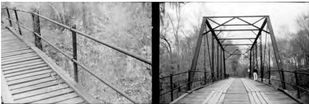
Figure 1. Two views of the Jennings Bridge over the Alapaha River, Hamilton County. This Pratt truss bridge was built from 1902-1903 by the American Bridge Company for $2,788. Source: State Archives of Florida, Florida Memory, http://floridamemory.com/items/show/139240 .
