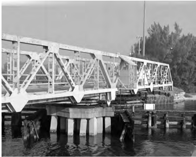
Figure 2. Blackburn Point Bridge in Sarasota County, a Warren pony truss swing built in 1925-1926 by the Champion Bridge Company. Source: State Archives of Florida, Florida Memory, http://floridamemory.com/items/show/139314 .
