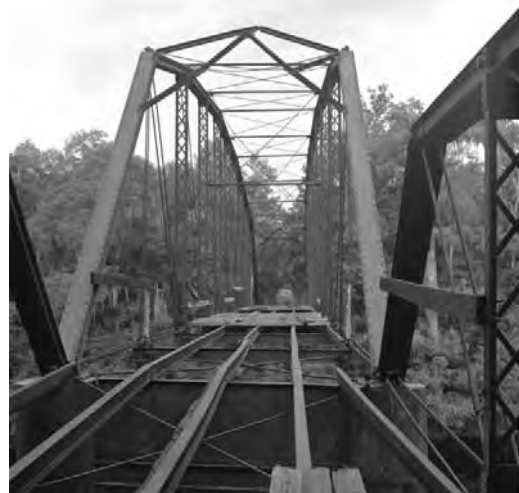
Figure 5. A camelback truss bridge over the Withlacoochee River, built in 1912 by the Converse Bridge Company at a cost of $4,297. Source: State Archives of Florida, Florida Memory, http://floridamemory.com/items/show/139262 .
