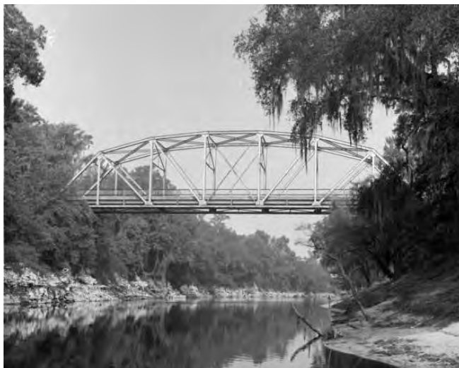
Figure 4. Suwannee Springs Bridge over the Suwannee River, Suwannee County. Parker through truss built in 1931 by the Austin Brothers Bridge Company of Atlanta. http://floridamemory.com/items/show/139253 .
