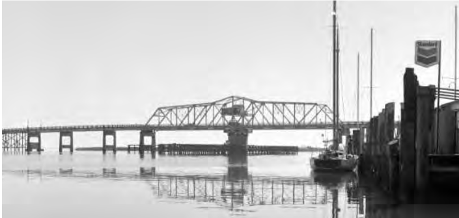
Figure 11. John Gorrie Bridge over Apalachicola Bay on US-98. This through truss swing bridge was built in 1936 and in use until 1989 when a new bridge was constructed.
