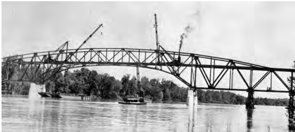
Figure12. Construction of the Blountstown Bridge over the Apalachicola River, 1937.
