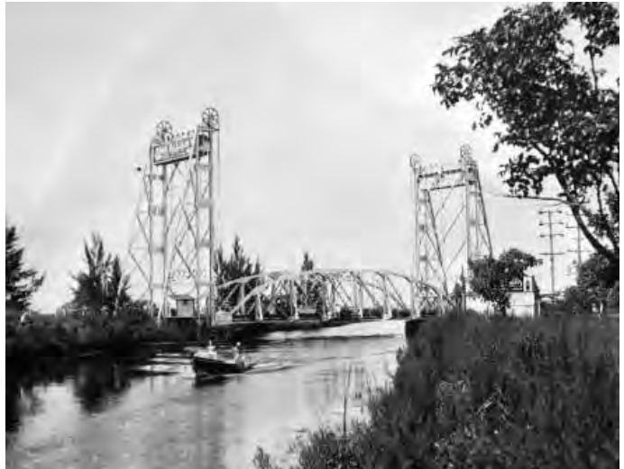
Figure 3. Vertical lift bridge built in 1928 by the Champion Bridge Company. Originally located at Northwest 36 th Street, and moved in 1954 to East First Avenue over the Miami Canal. Source: State Archives of Florida, Florida Memory, http://floridamemory.com/items/show/138120 .
