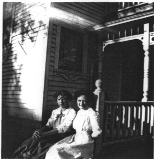
Date of photo: 1910 SW corner and south porch
