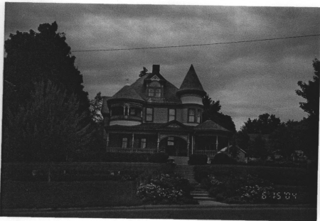
Figure 1: 1706 Broadway (in tact and well maintained, rating of 10).
