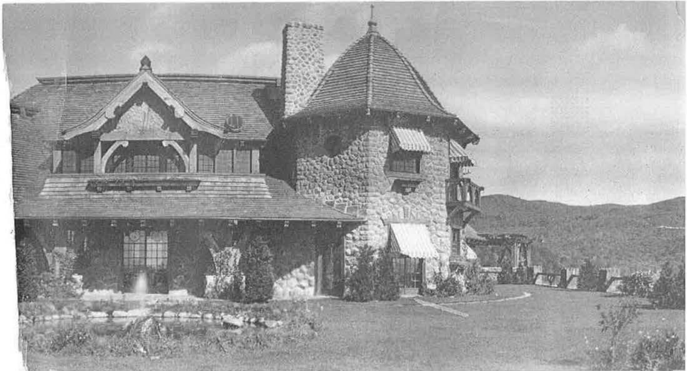
Fig. 16: Lakeside elevation, showing the dining room/master bedroom turret and terrace pool. From Olive D. Plant photo album.
