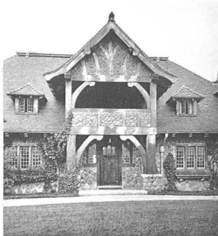
Fig. 19: Front entrance to house, showing the extensive use of local materials crafted by artisan workers. From "For Sale....." (1924 Sales Booklet).
