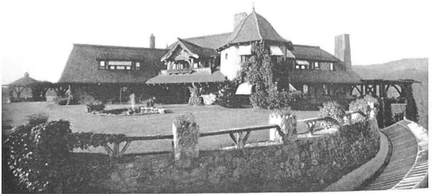
Fig. 15: Lakeside elevation of house and the terrace, the only formal landscape on the property. The roof of the greenhouse is visible in the foreground at far right. From "For Sale....." (1924 Sales Booklet).
