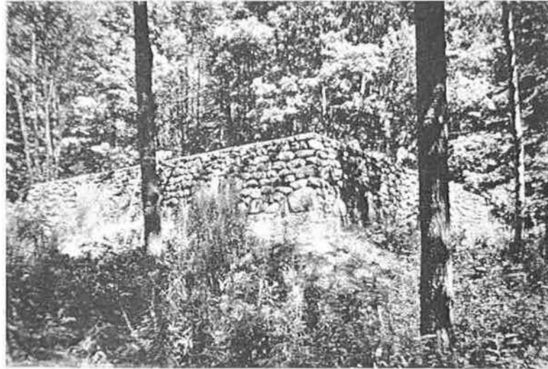
Fig. 9: Main Reservoir. This reservoir, one of two on the nominated property and built of local stone, served Plant's house and stable/garage, as well as the two lodges.
