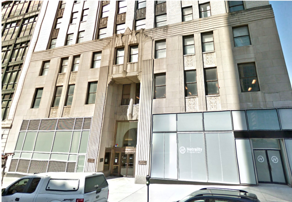
Figure 21 – Bryant Building, 1102 Grand Avenue (Google Maps 2017)
