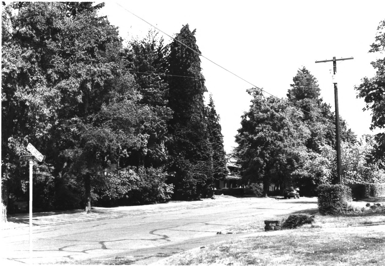
1 Pennsylvania Ave - W. Side H.D., Chehalis, Lewis Co., WA Photo #1
