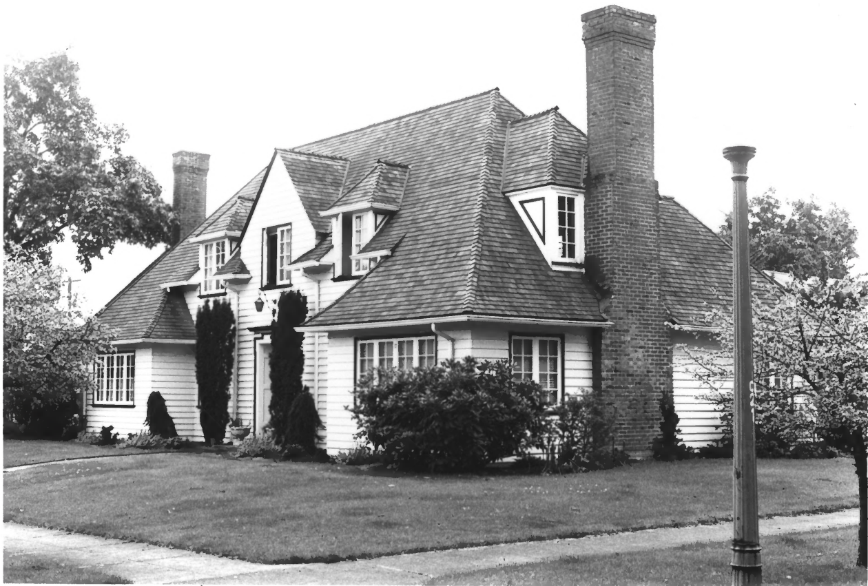
Pennsylvania Avenue - W. Side H.P., Chehalis, Lewis Co., Photo 25
