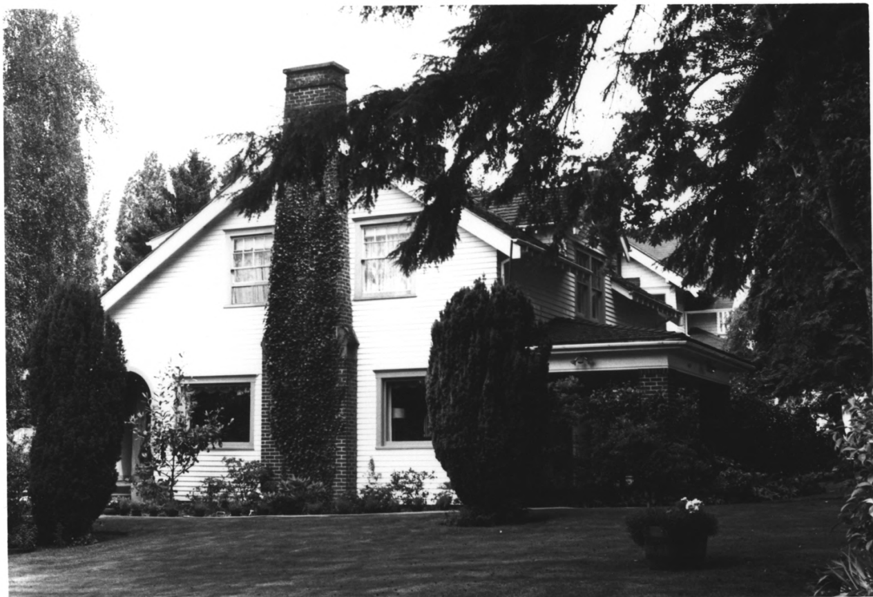
Pennsylvania Ave - W. Side H.D., Chehalis, Lewis Co., WA Photo #2
