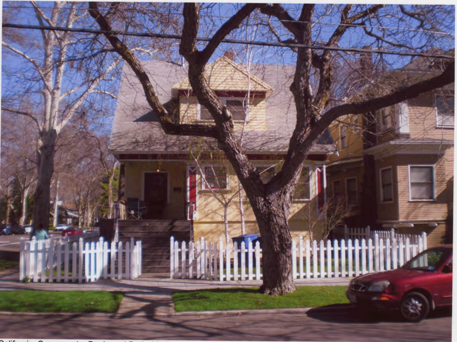
California_Sacramento_Boulevard Park_0017 Eugene Hepting House, Colonial Revival residence, 501 22 nd Street, facing east
