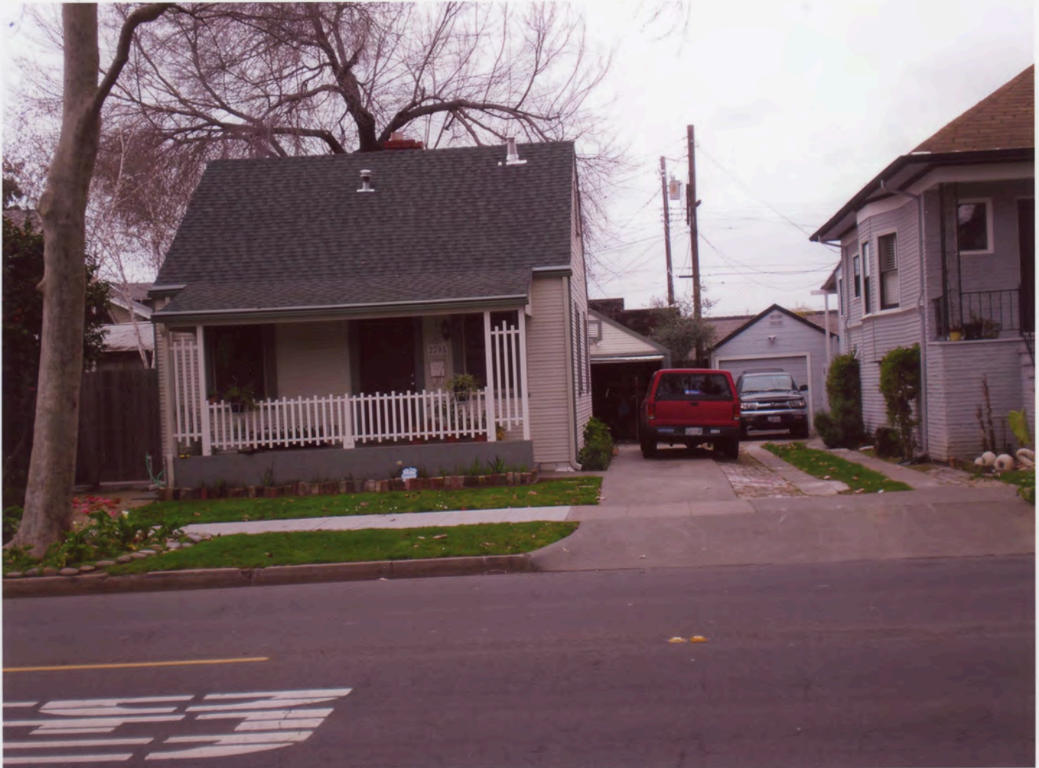
California_Sacramento_Boulevard Park_0010 Minimal Traditional cottage, 2205 C Street, facing north
