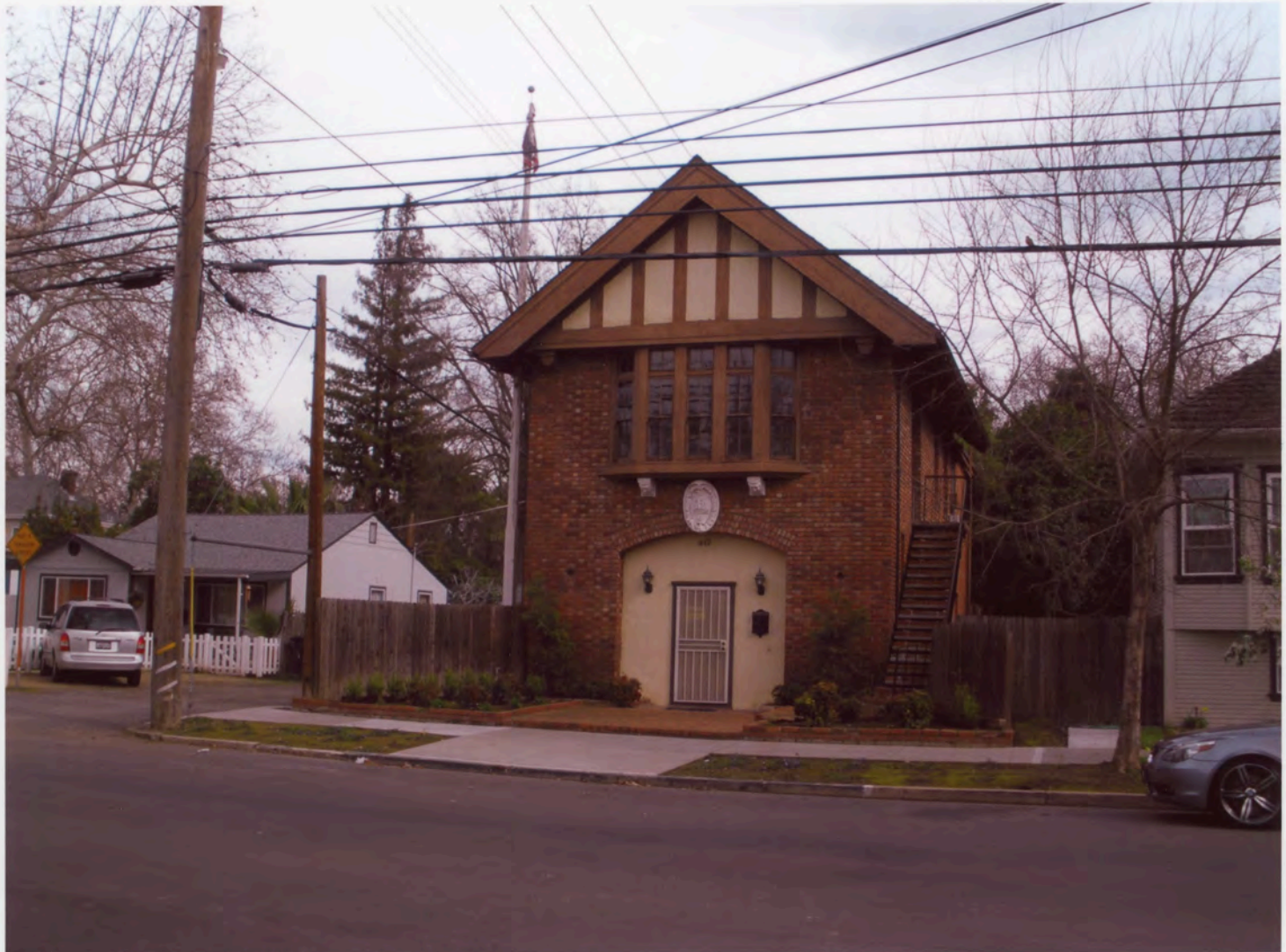
California_Sacramento_Boulevard Park_0005 Sacramento Fire Department Station #4, 417 20 th Street, facing east
