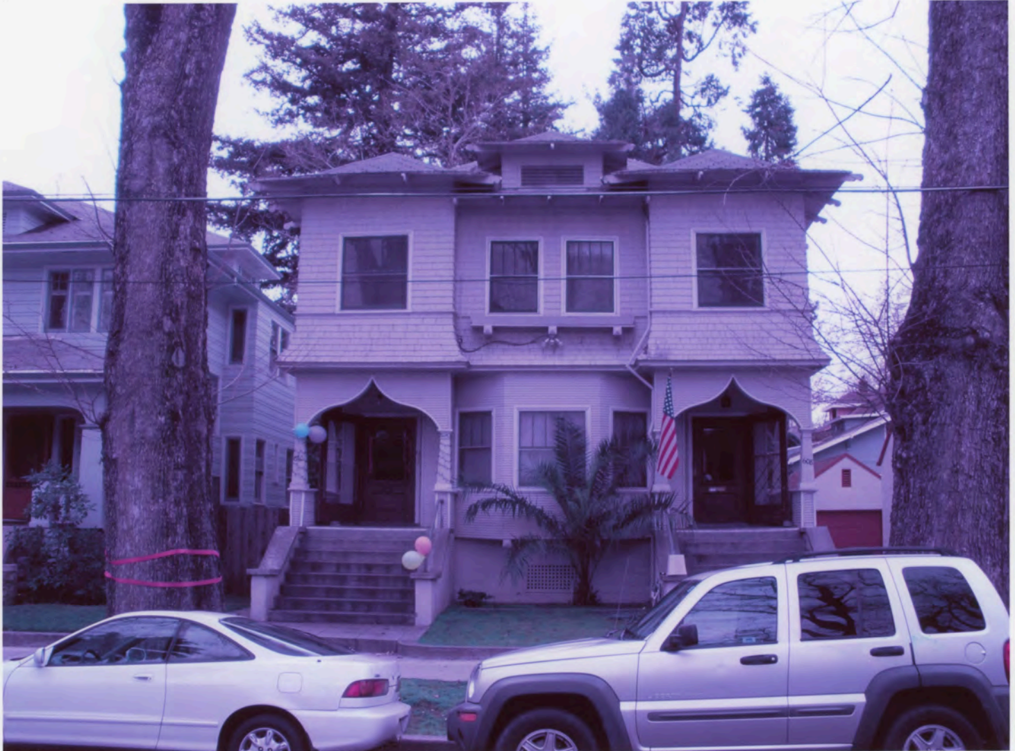
California_Sacramento_Boulevard Park_0008 Clarence Smith House, Asian influenced Craftsman duplex, 608-610 21 st Street, facing west
