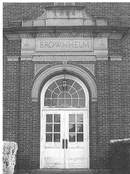
Figure #27 Brownhelm School doorway, Lorain County, by Fulton, Taylor and Cahill in 1922 ( http://www.oldohioschools.com/portage_county.htm )
