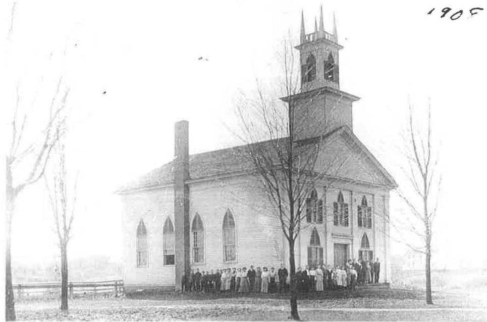
Figure #9 Historic photograph of Mantua Center Methodist Church, looking southwest
