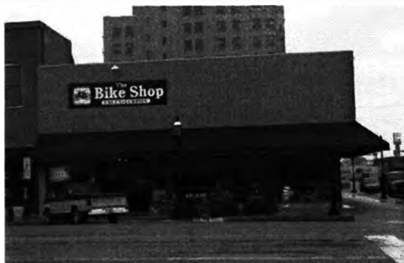
Photo 43. 202-204 W. Randolph Avenue, 1950s Commercial Building
