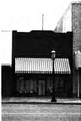
Photo 94. 113 S. Grand Avenue, One-Story Commercial Style
