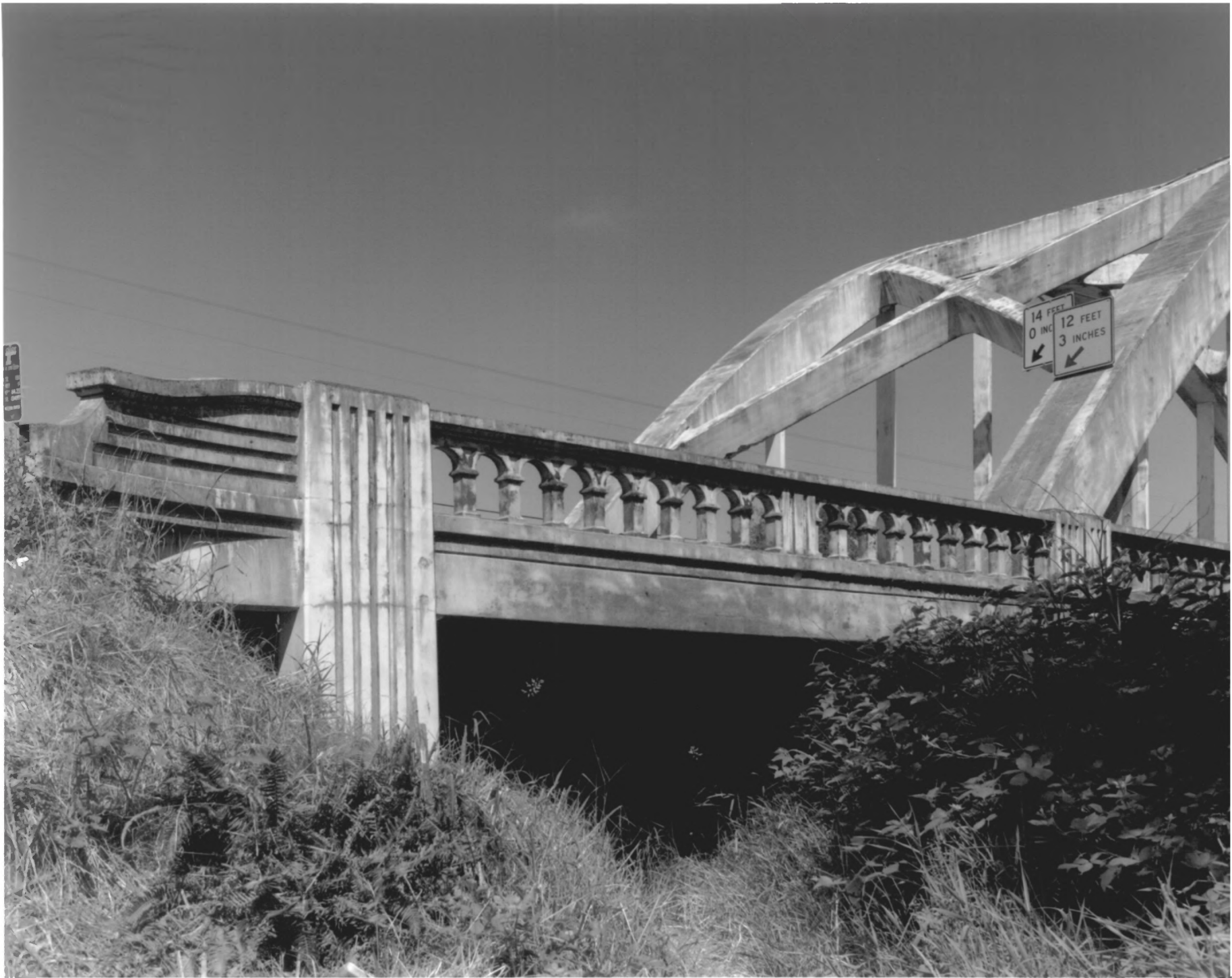
WILSON RIVER BRIDGE, TILLAMOOK, OREGON
