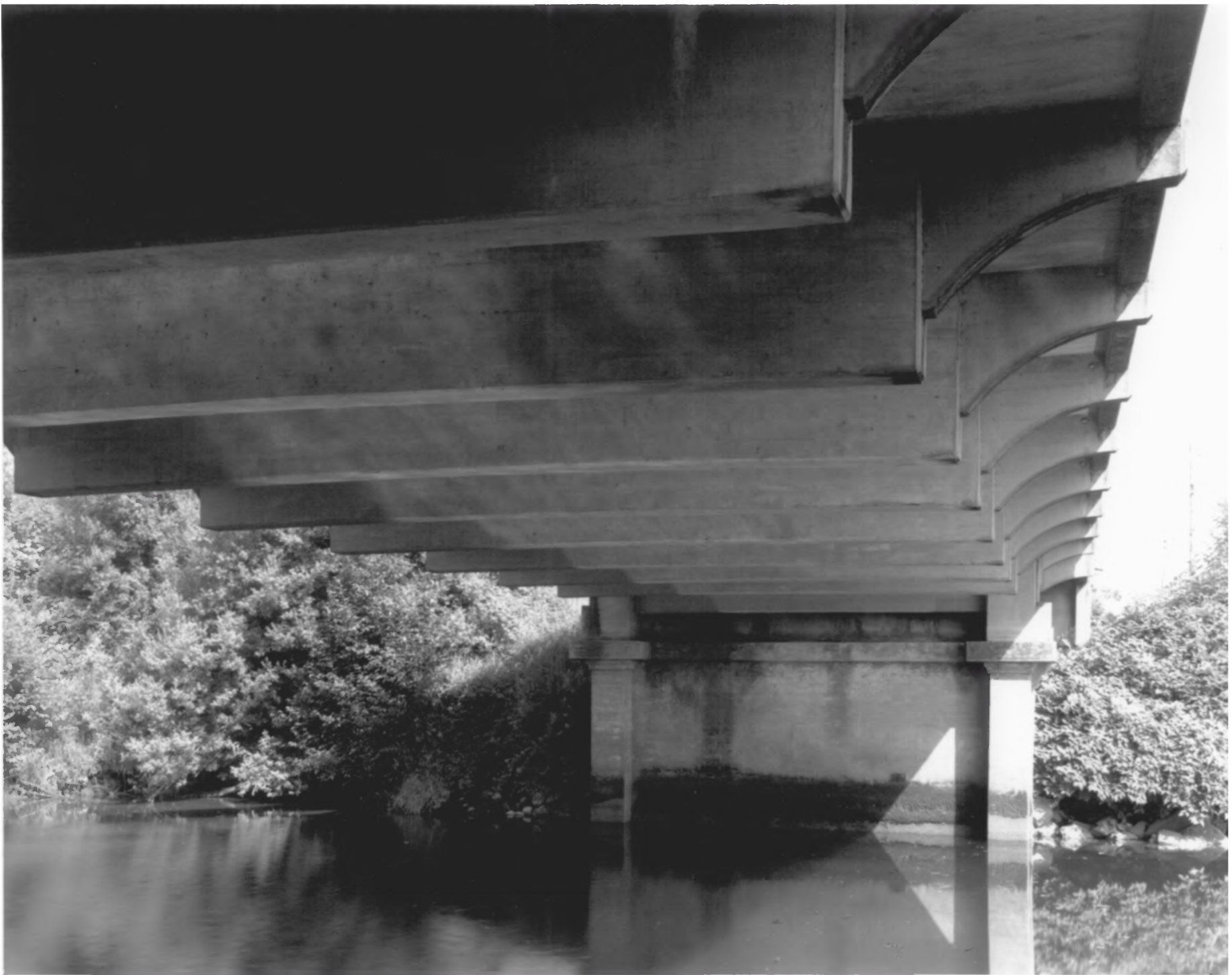
WILSON RIVER BRIDGE, TILLAMOOK, OREGON
