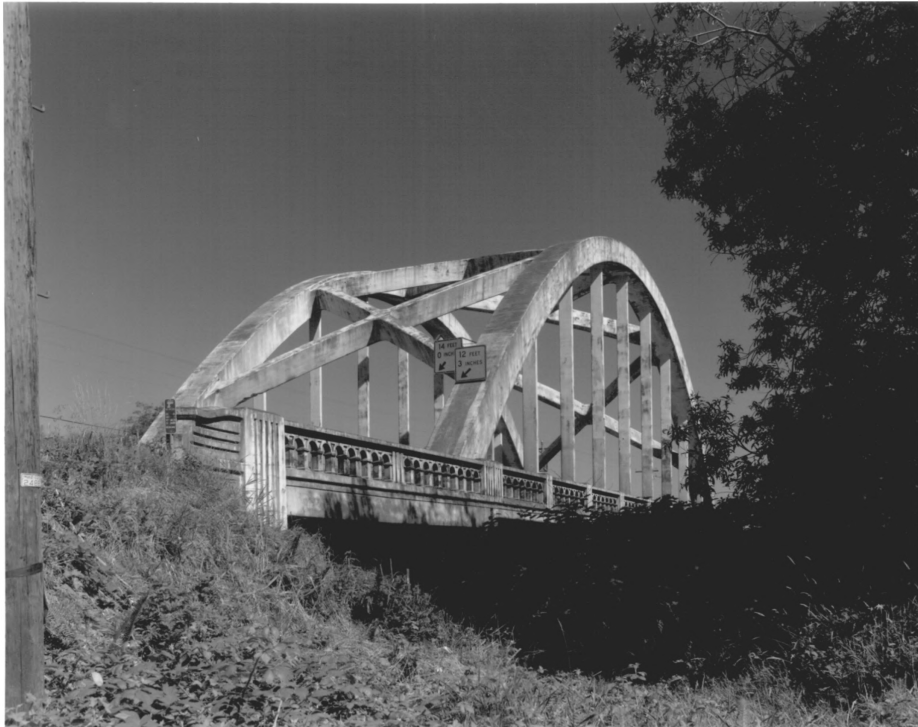
WILSON RIVER BRIDGE, TILLAMOOK, OREGON #2
