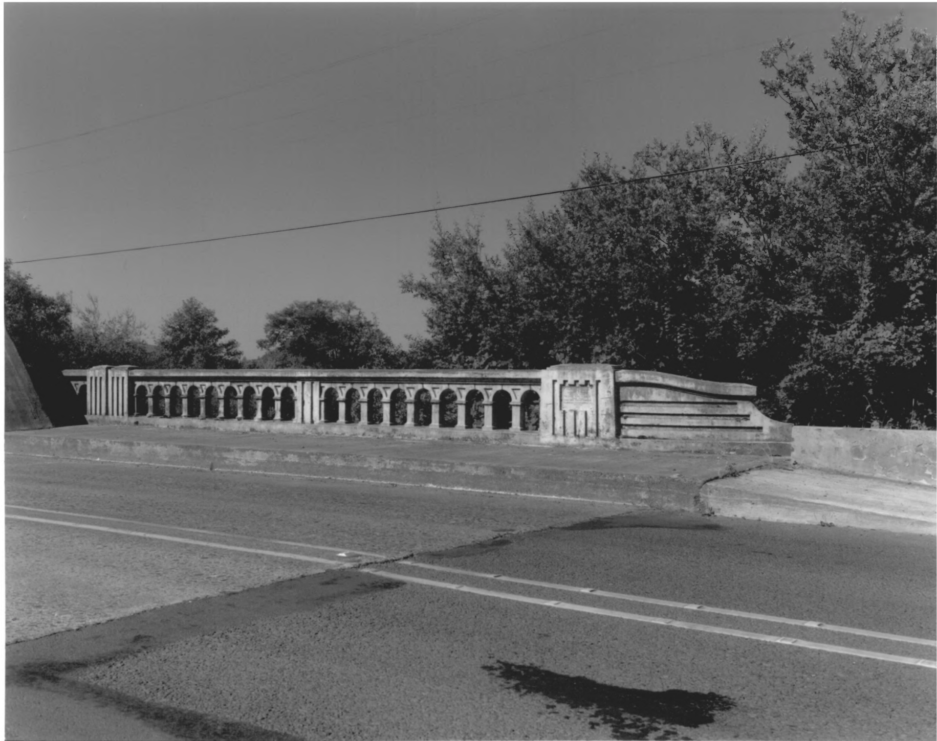
WILSON RIVER BRIDGE, TILLAMOOK, OREGON
