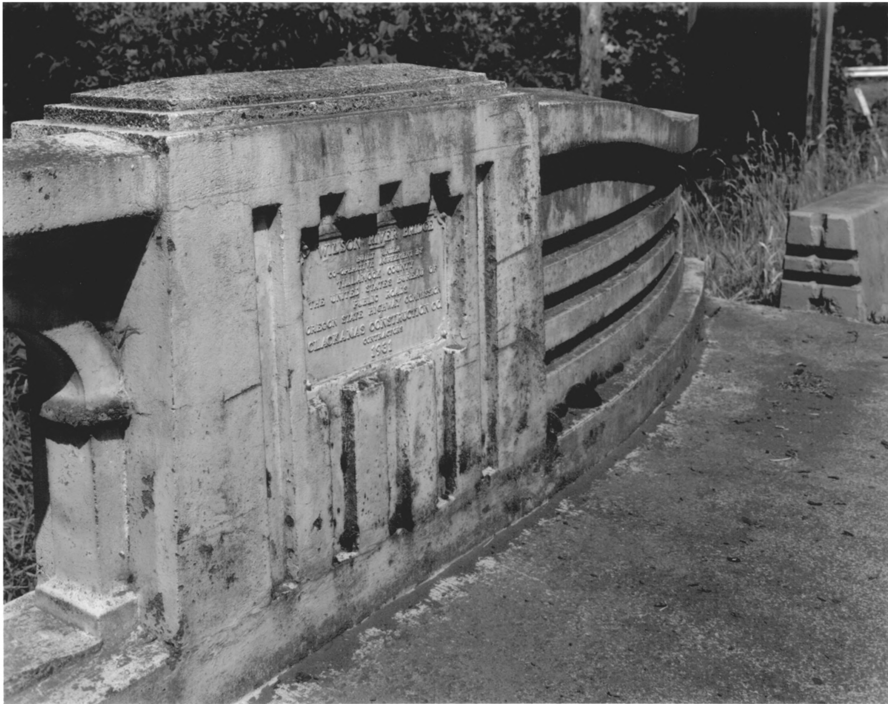
Wilson River Bridge, Tillamook, Oregon
