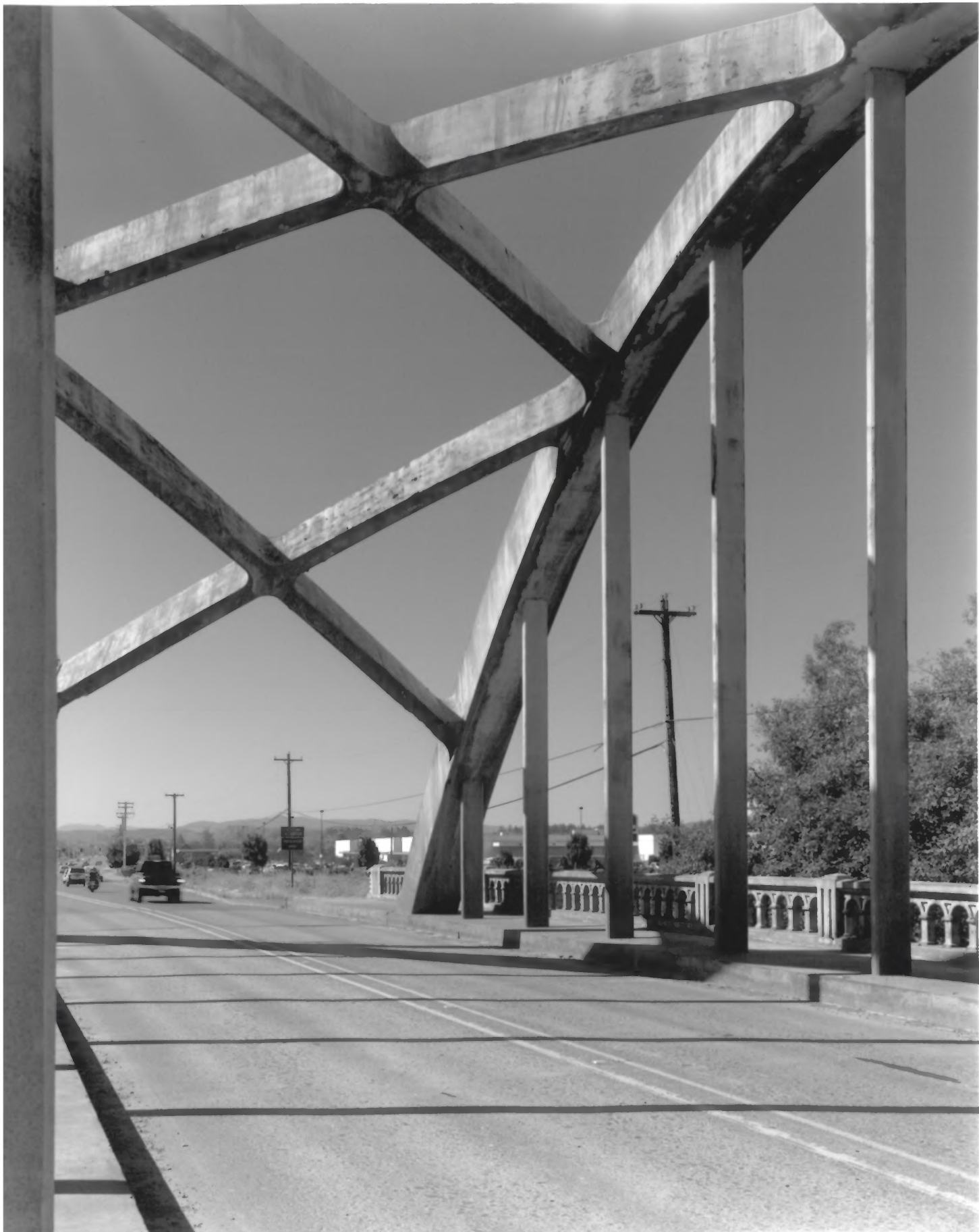
WILSON RIVER BRIDGE, TILLAMOOK, OREGON # 1
