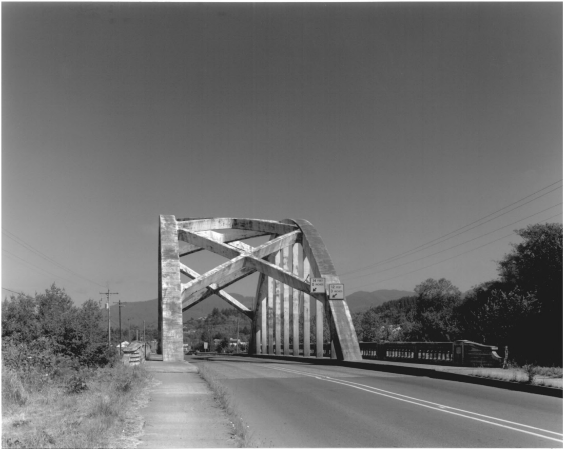
WILSON RIVER BRIDGE, TILLAMOOK, OREGON # 3
