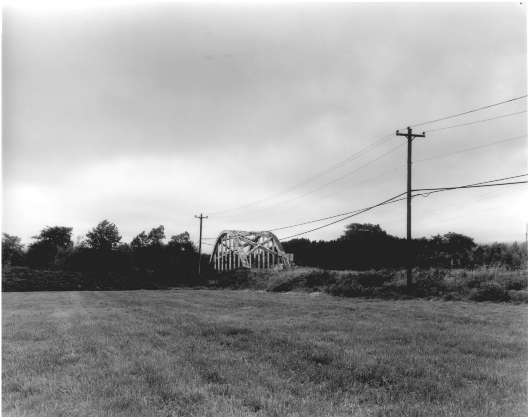
WILSON RIVER BRIDGE, TILLAMOOK, OREGON
