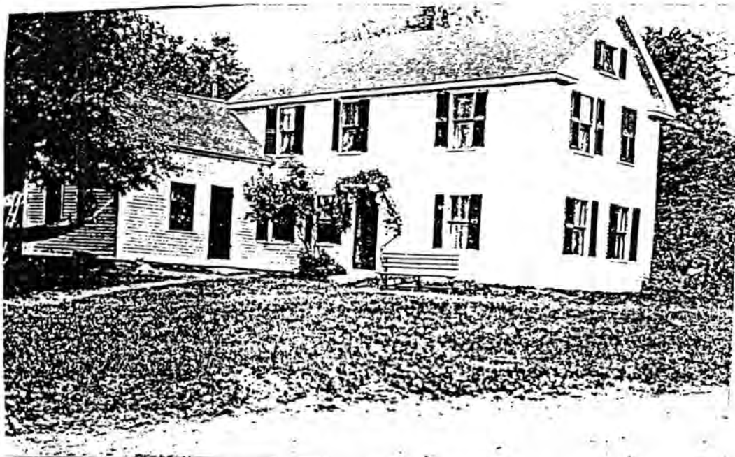
Ⓑ 146 WICKABOAG VALLEY ROAD AFTER ALTERATIONS MADE BY THE DUNCANSONS, NOTE BROAD EAVES AND GABLE RETURNS. (PHOTOGRAPH WEST BROOKFIELD HISTORICAL COMMISSION)
