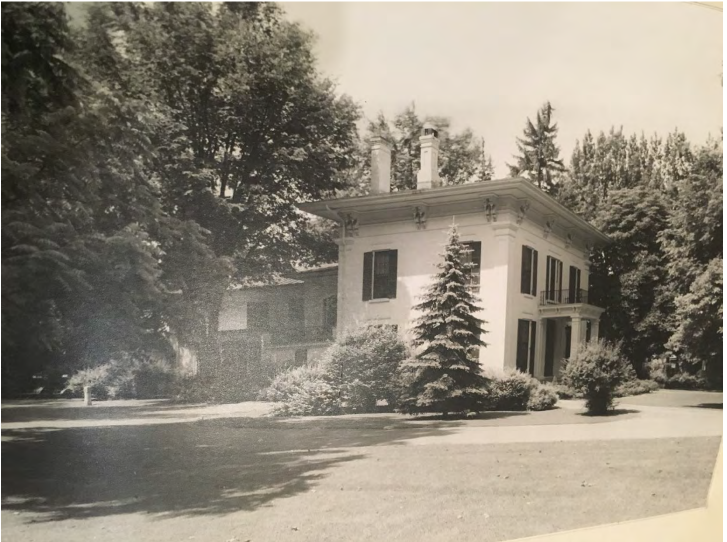
Building at 53 West Main Street (1940)
