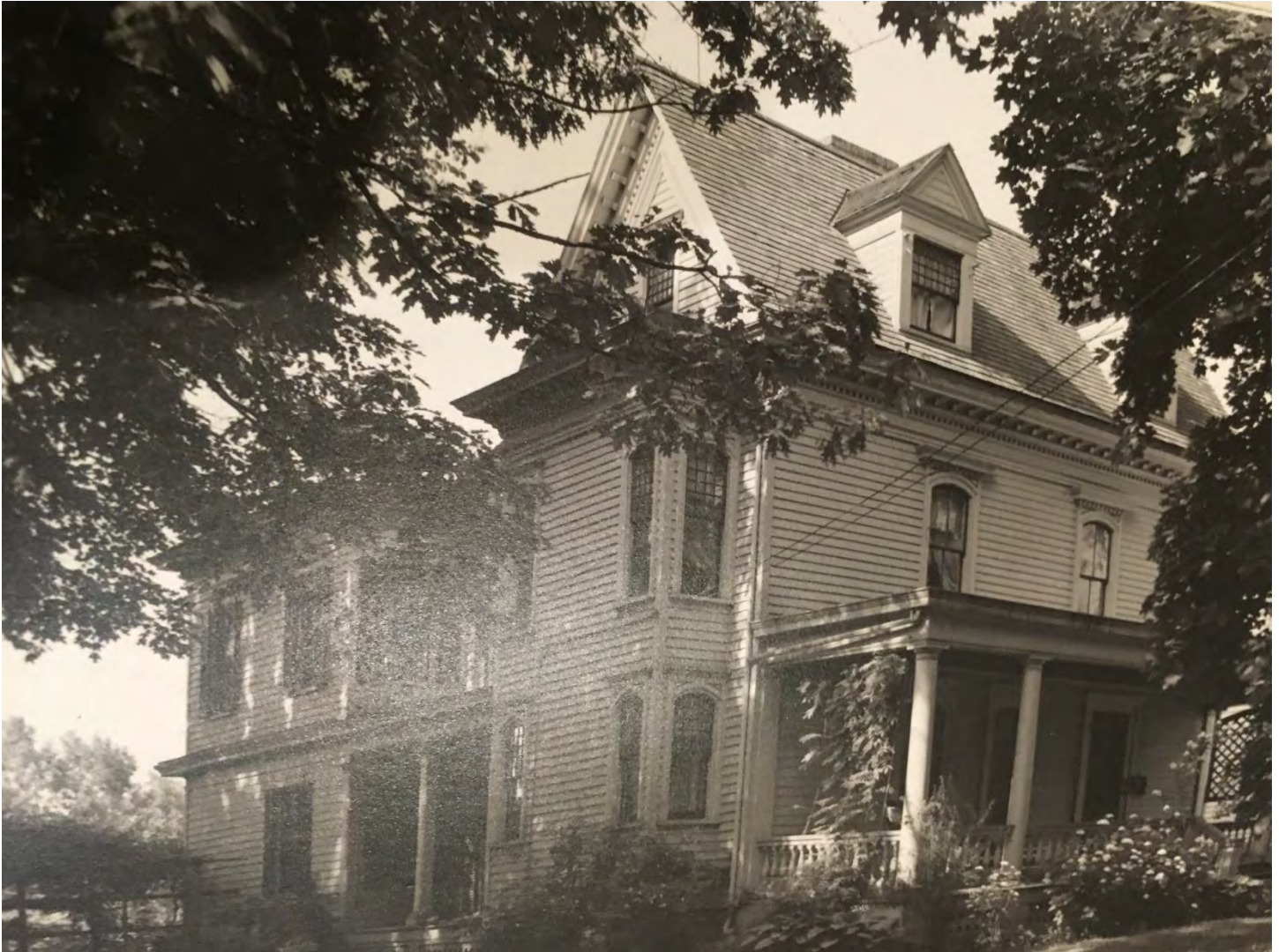
Residence at 29 West Main Street (1940)
