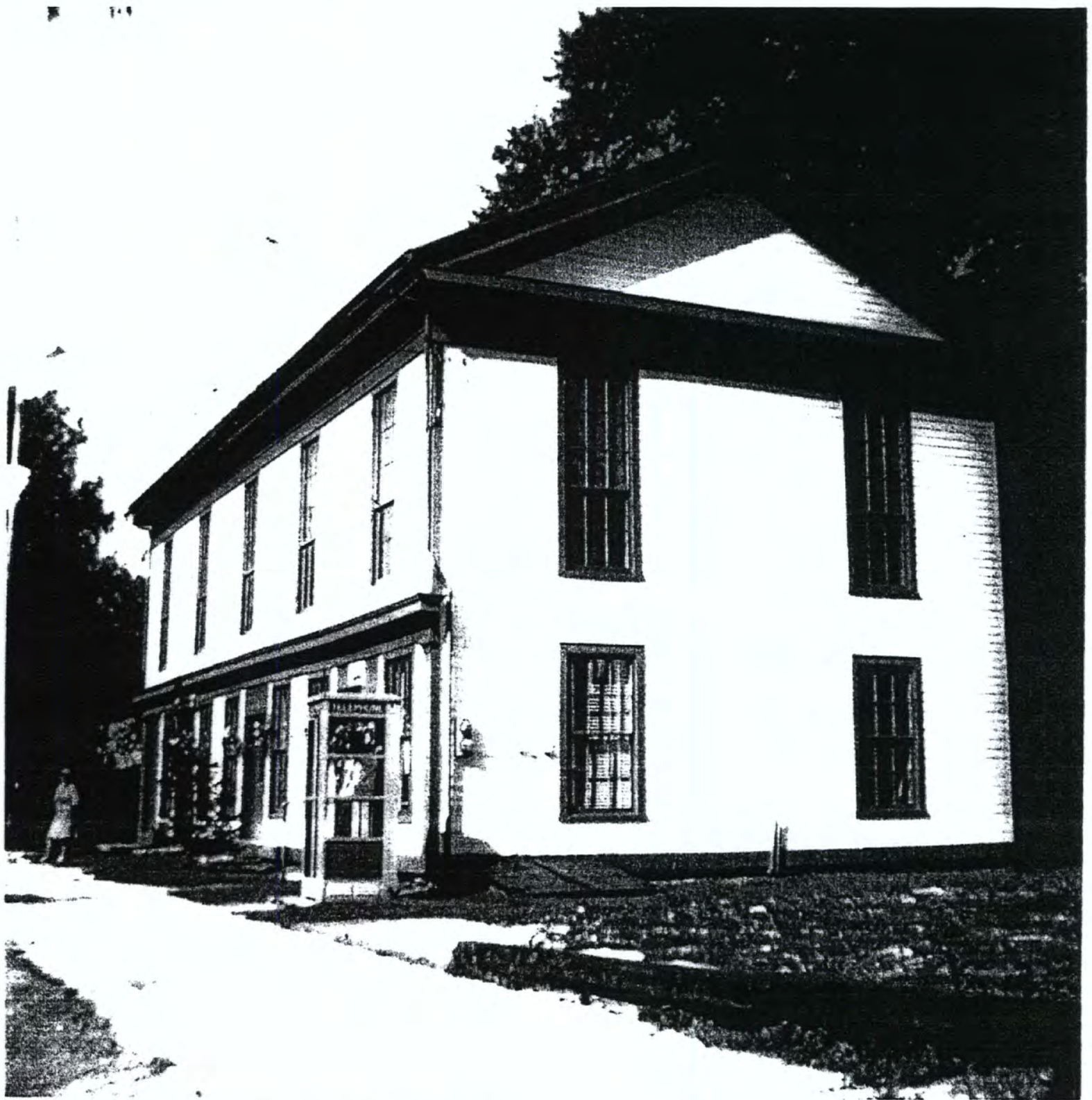
West Stockbridge Town Hall, 1970s From West Stockbridge Folder (W-4), 697-706, Berkshire Historical Photograph Collection, Berkshire County Historical Society.
