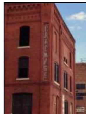
deteriorated north addition was removed and is being reconstructed. A new bay of windows is being introduced on the west side. More challenging to the historic character of the buildings will be the addition of residential stories above the original structures, set back from the street facades. When the work is completed, the historic integrity of 818 and 808 Q Streets as "contributing" properties should be evaluated.
