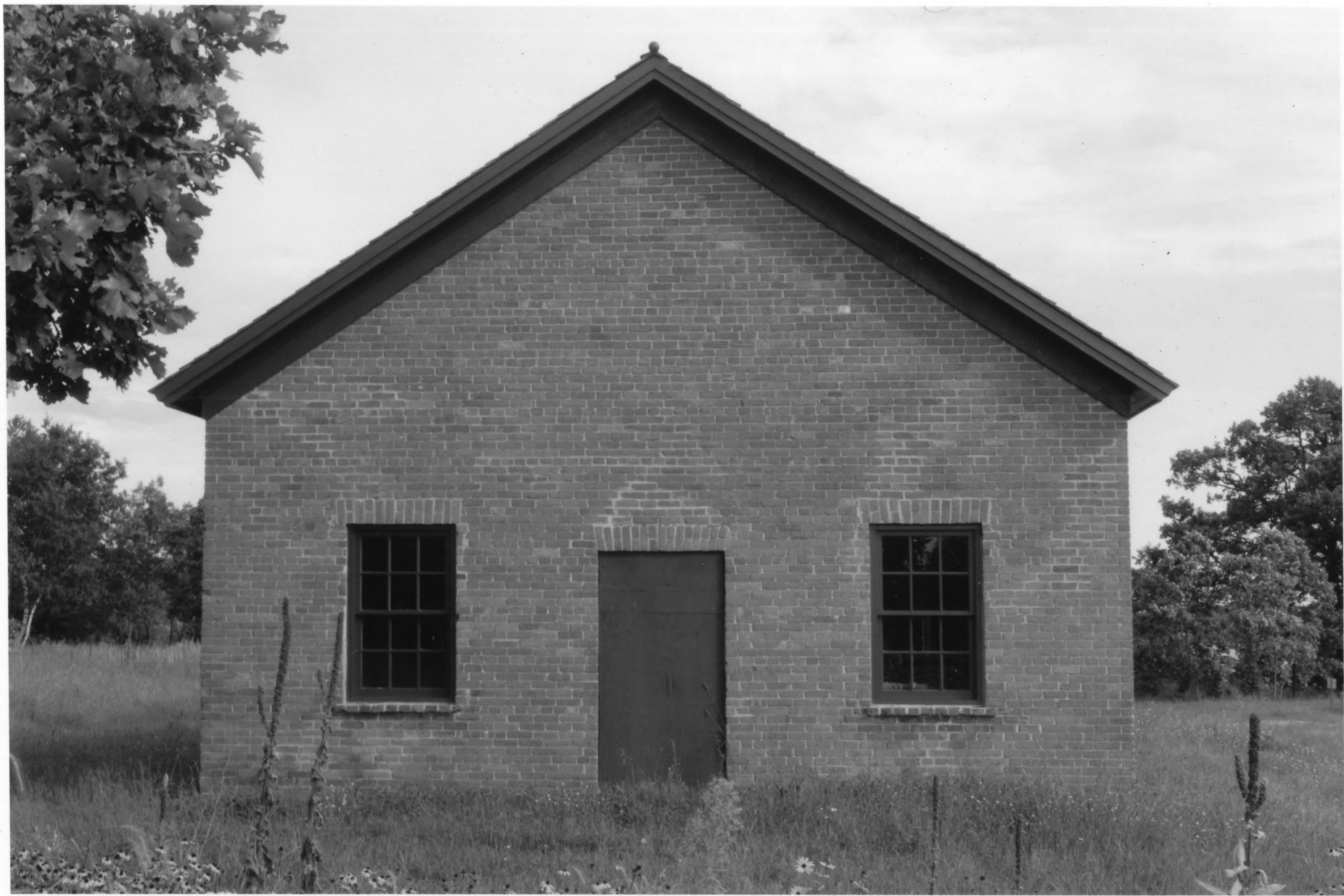
DAIRY Building, GRANARY, Root Cellar and auxiliary buildings, NORTH OAKS FARM, NORTH OAKS Ramsey CO., MN 013270-12
