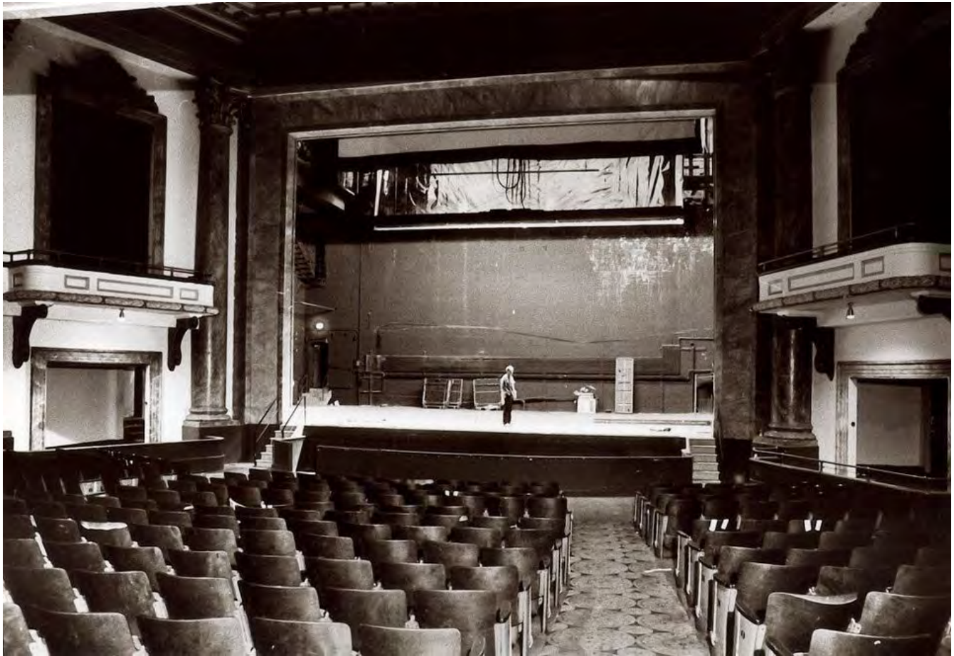
Figure 9: Interior of WHK Studio One theatre (Metropolitan Theatre). Date Unknown
