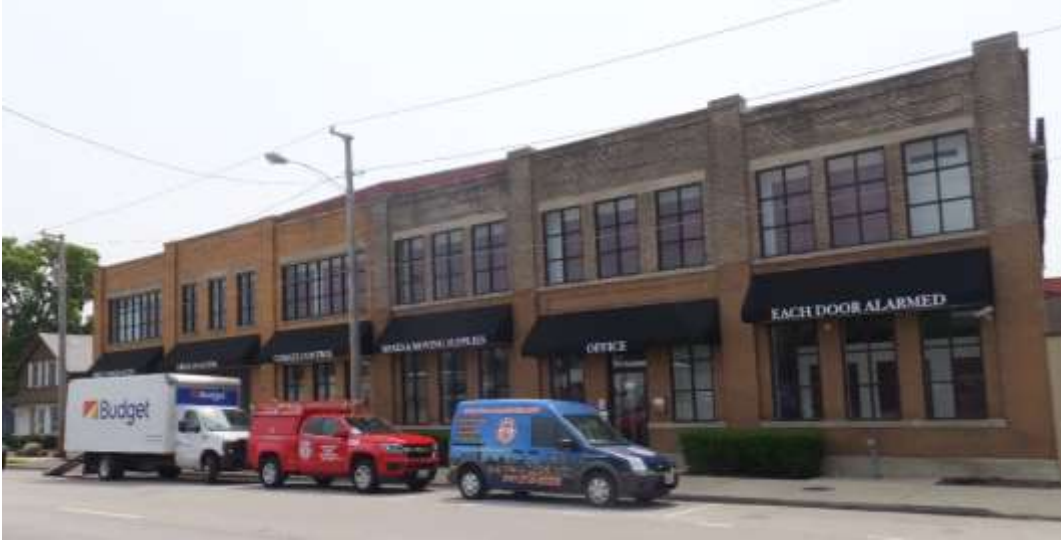
Fig. 17 – Current view of 232 S. Lake St. – West elevation
