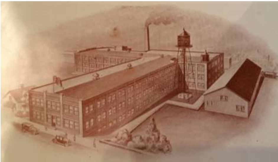
Fig. 16 – Rendering of the Pictorial Printing factory illustrating 2 nd floor addition and warehouse Pictorial Packages: First Aid to More and Better Business , 1925
