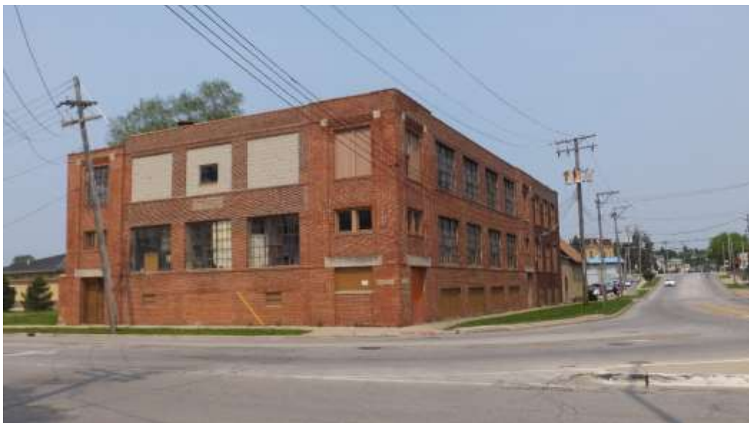
Fig. 4 – Current view of 301 S. River St. – East and North elevations
