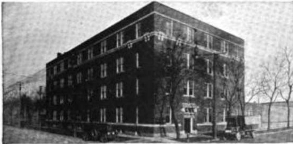
Fig. 8 – Photo of the new International Harvester building at S. River and Gale Streets. Harvester World, Vol. 3-4, 1912
