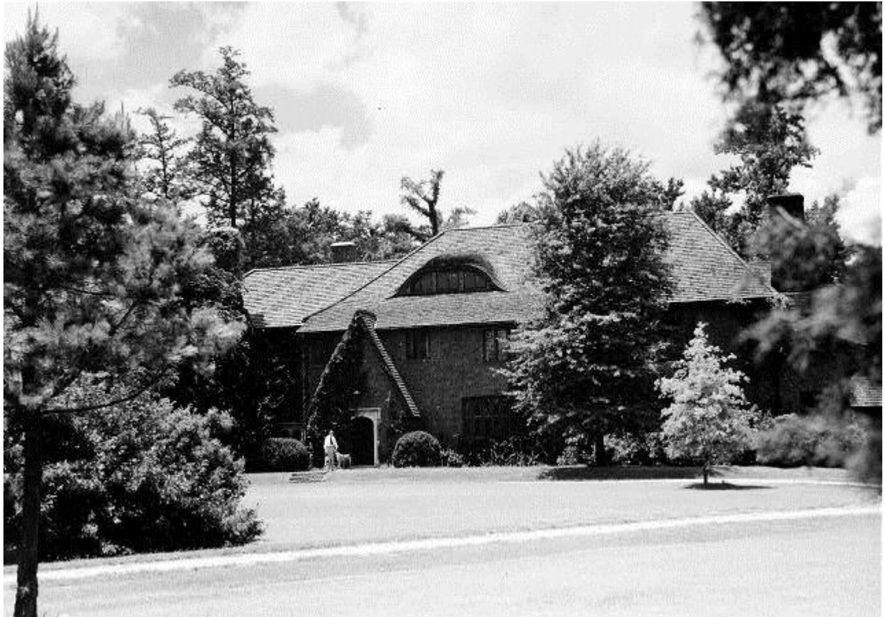
Figure 6: Robert (Roy) E. L. Wilson House, 1939 (Photo courtesy Arkansas History Commission)
