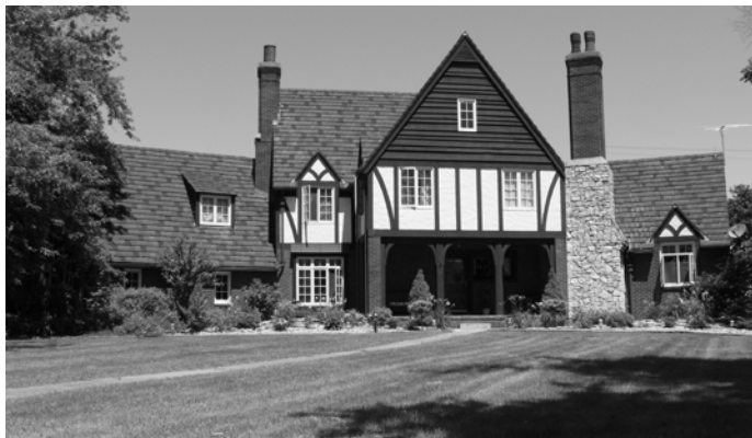
Figure OO Truit House (1940). Private photograph.
