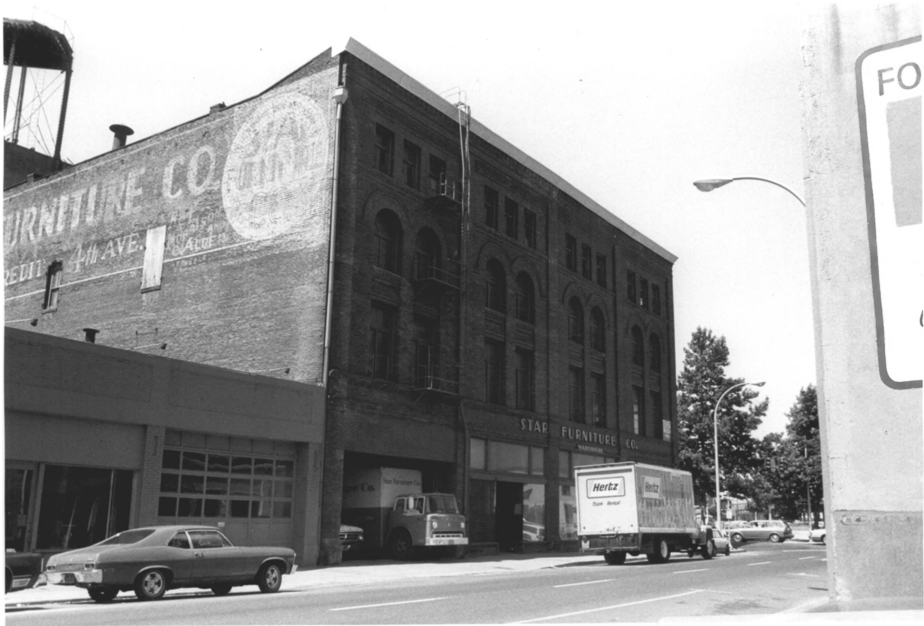
View of east elevation of Oregon Cracker Company Building AUG 14 1979
