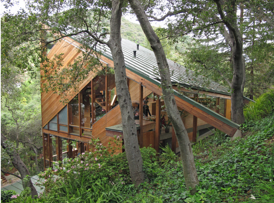
View of west and south façades. (Photo credit: Shelly White, date of photograph unknown)
