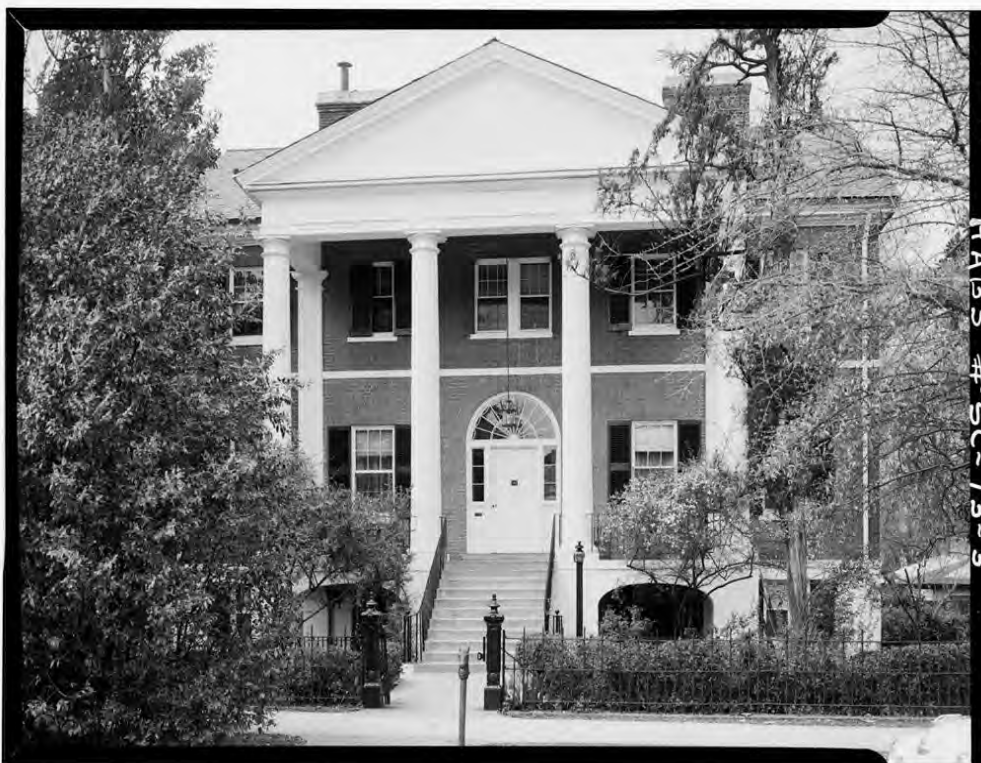
Figure 6: Historic American Buildings Survey, April, 1960 Front (South) Elevation, 1401 Laurel Street, Columbia, Richland County, S.C.
