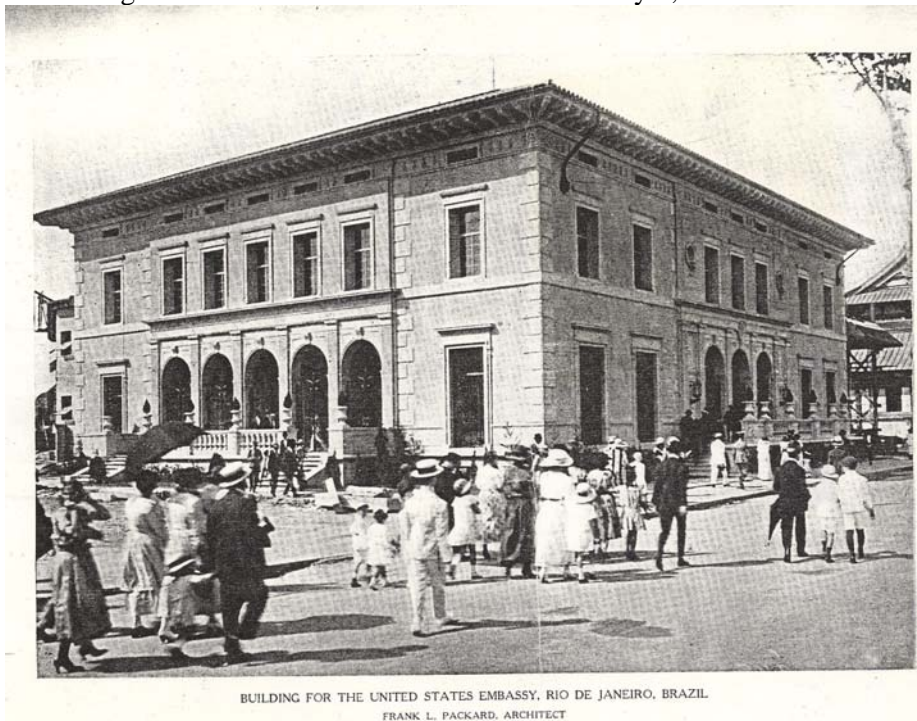
Figure 11. Ca. 1925 photograph of the United States Embassy building in Rio de Janeiro, Brazil. Source: Provided by Barb Powers, Department Head, Inventory & Registration, OHPO, April 29, 2014.
