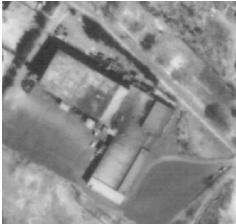
Fig. 6 Rochambeau Worsted Company Mill, 1972 (Aerial Photographs of Providence, RI at http://www.mapper.provplan.org/ha/ )
