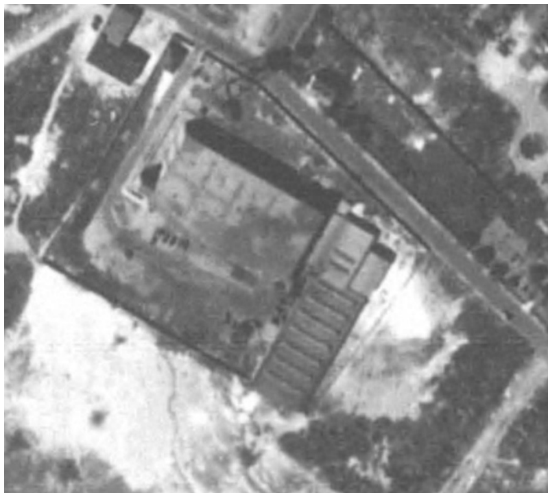
Fig. 3 Rochambeau Worsted Company Mill, 1939 (Aerial Photographs of Providence, RI at http://www.mapper.provplan.org/ha/ )
