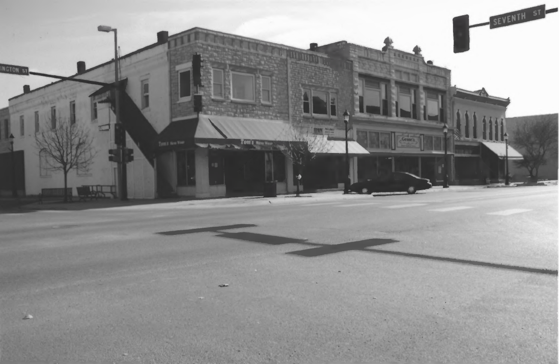
Junction City Downtown District, Geary County, Kansas #22
