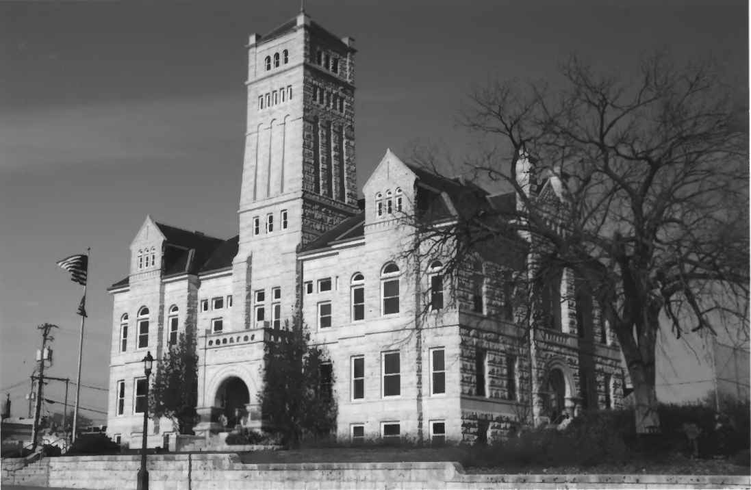
Junction City Downtown District, Geary County, Kansas #16
