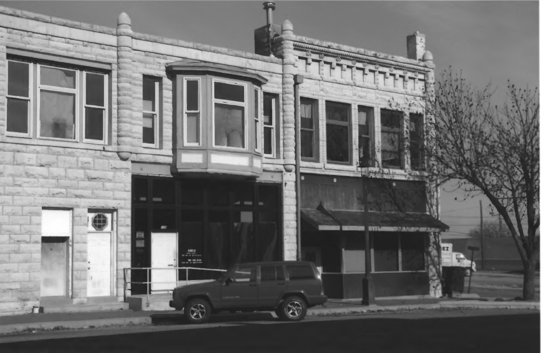
Junction City Downtown District, Geary County, Kansas #20
