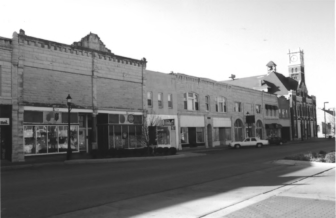
Junction City Downtown District, Geary County, Kansas
