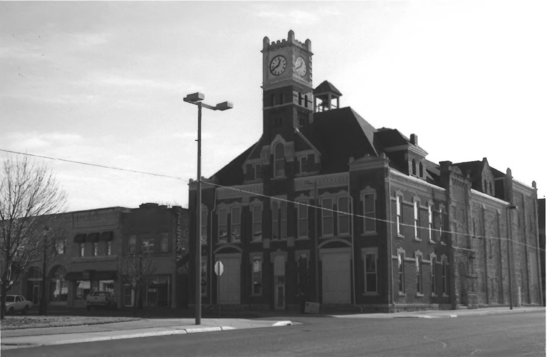
Junction City Downtown District, Geary County, Kansas #5
