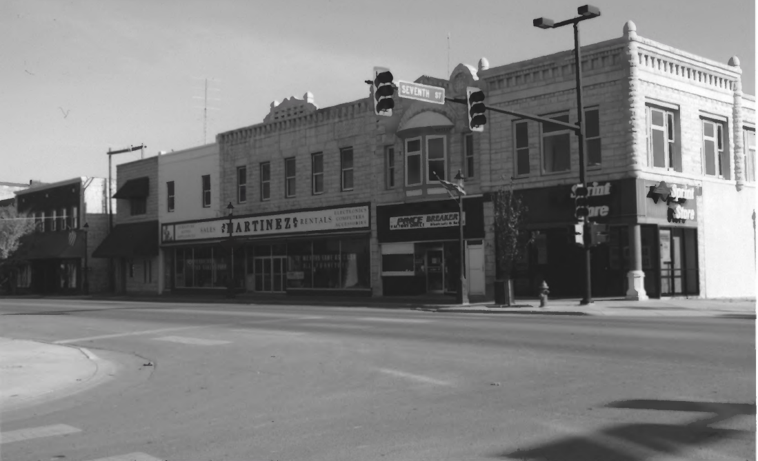
Junction City Downtown District, Geary County, Kansas #19
