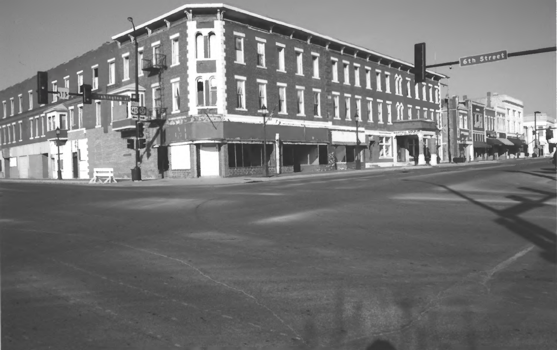
Junction City Downtown District, Geary County, Kansas
