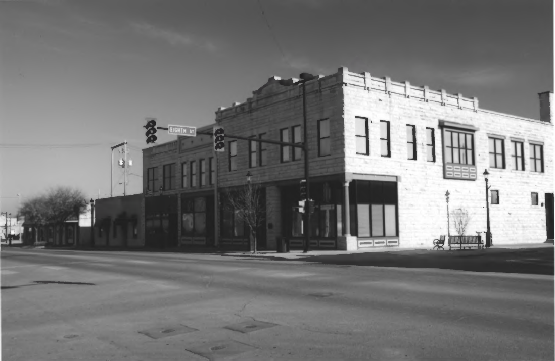
Junction City Downtown District, Geary County, Kansas
