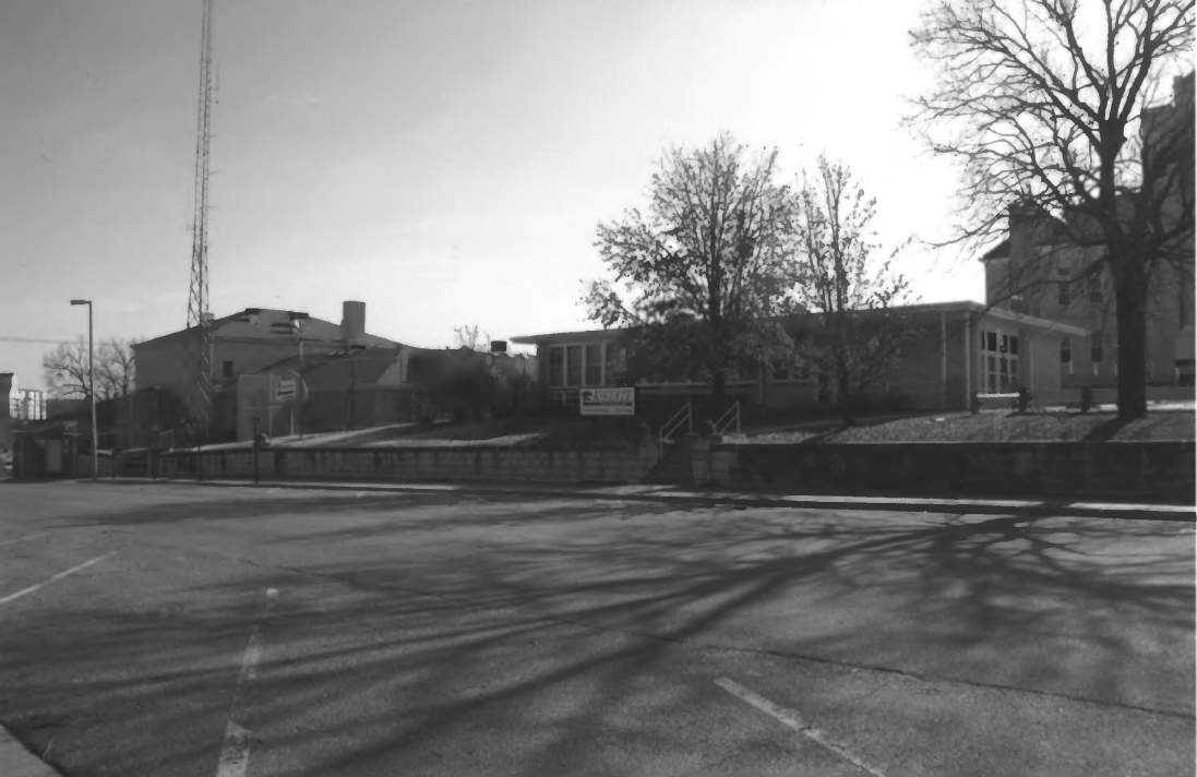
Junction City Downtown District, Geary County, Kansas #17
