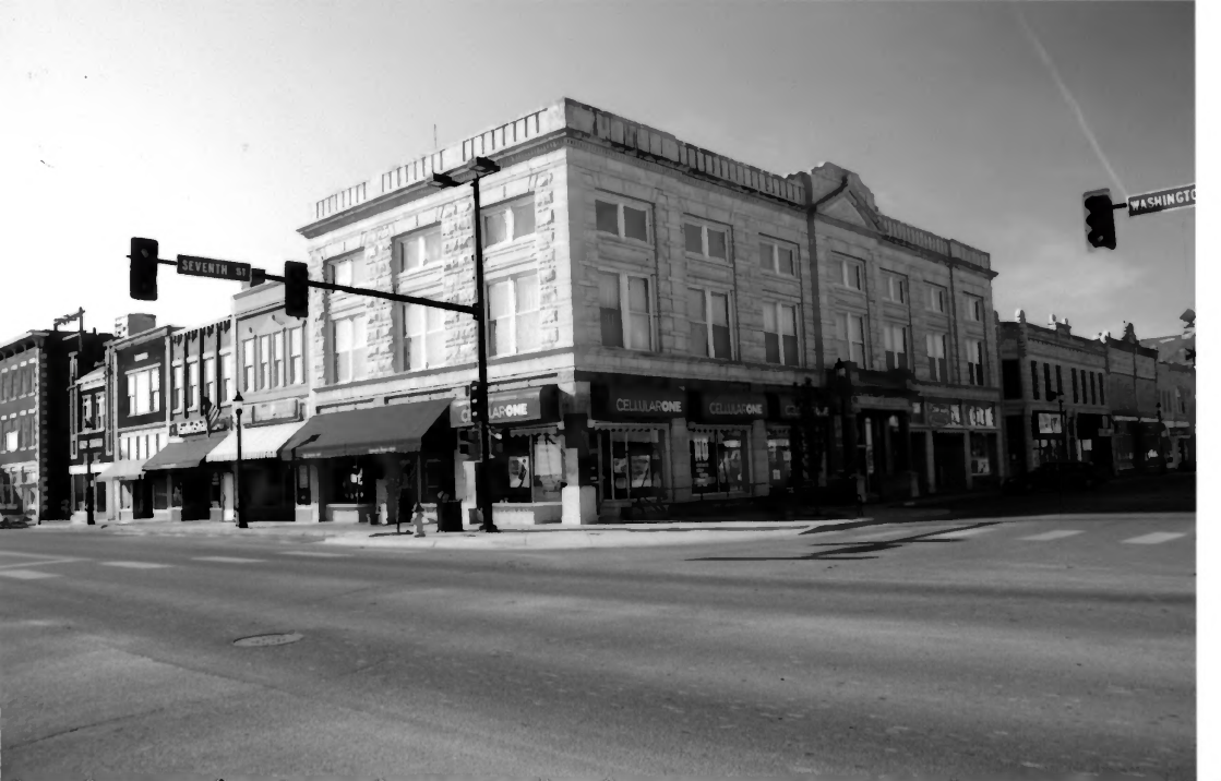
Junction City Downtown District, Geary County, Kansas
