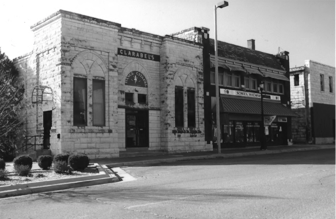
Junction City Downtown District, Geary County, Kansas #21
