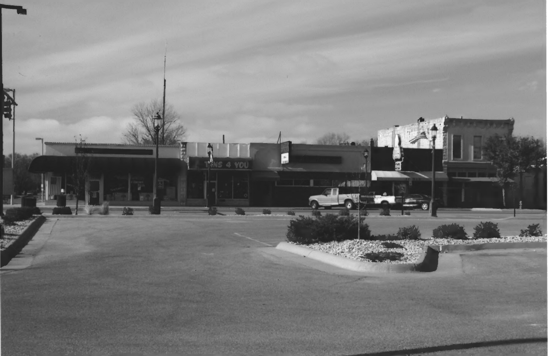
Junction City Downtown District, Geary County, Kansas #13
