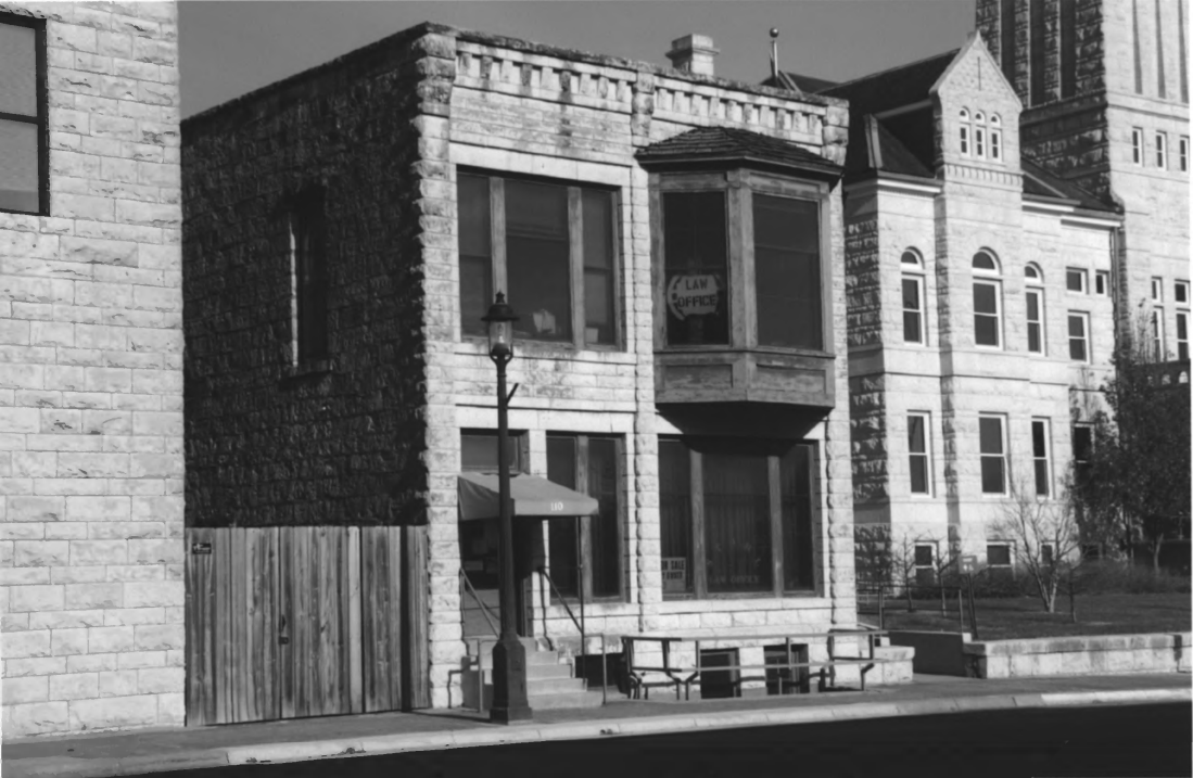
Junction City downtown District. Geary County, Kansas #15
