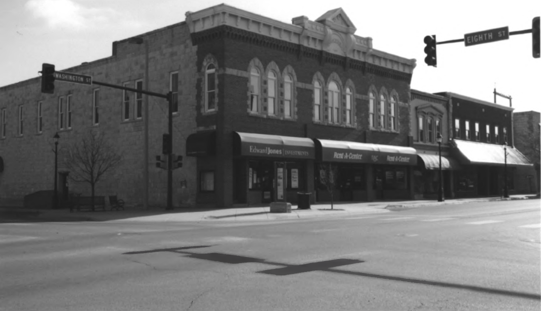
Junction City Downtown District, Geary County, Kansas
