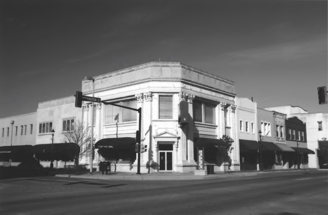
Junction City Downtown District, Geary County, Kansas #8
