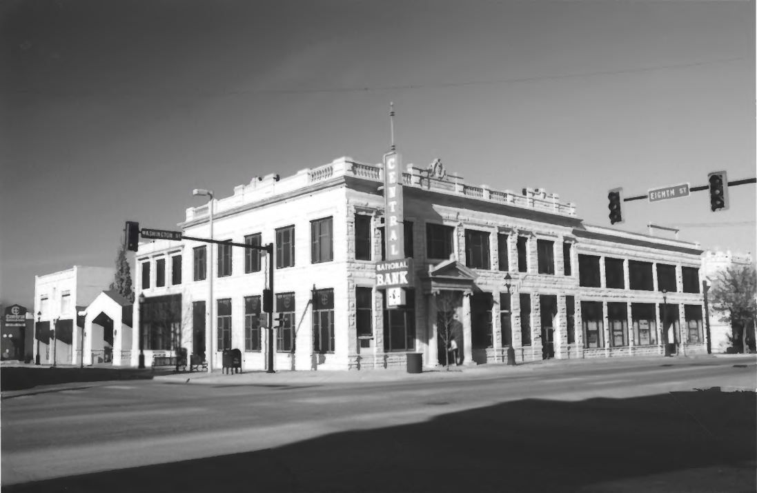
Junction City Downtown District, Geary County, Kansas
