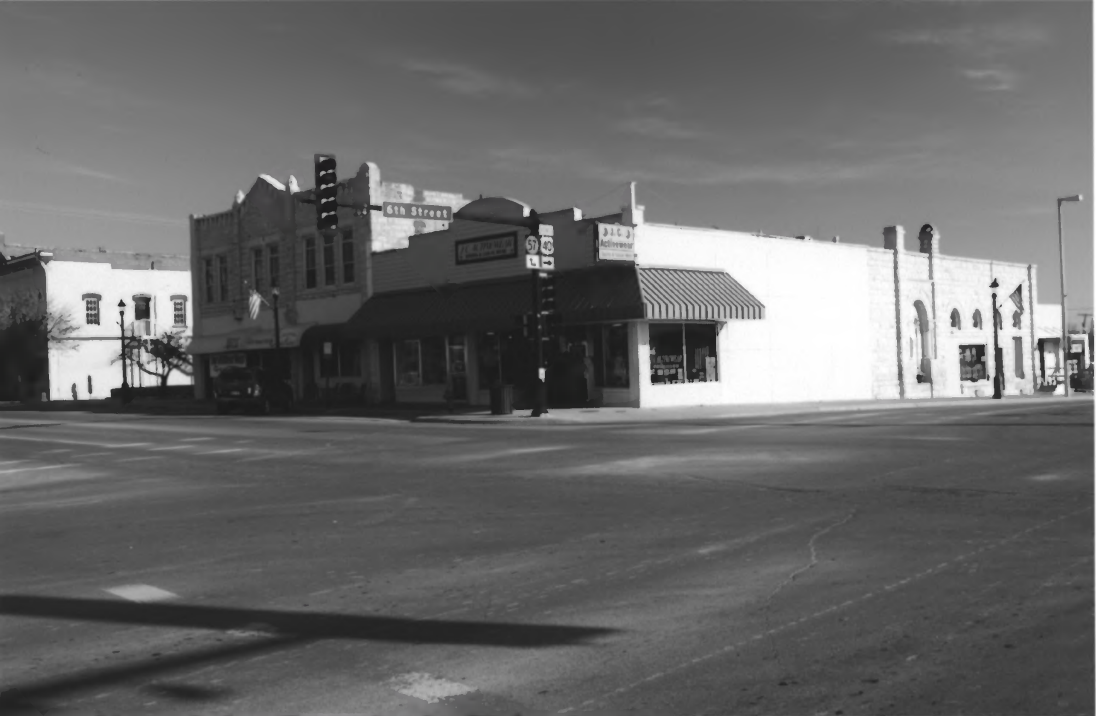
Junction City Downtown District, Geary County, Kansas #23
