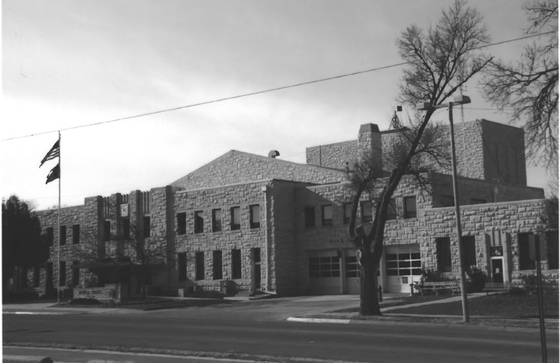
Junction City Downtown District, Geary County, Kansas
