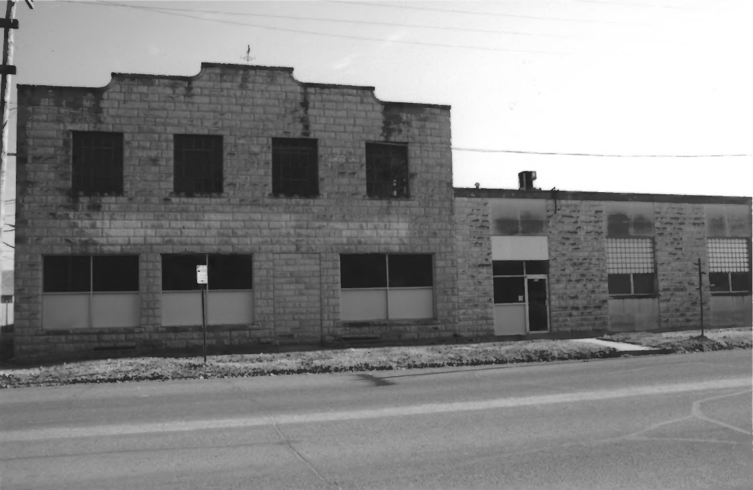
Junction City Downtown District, Geary County, Kansas #12
