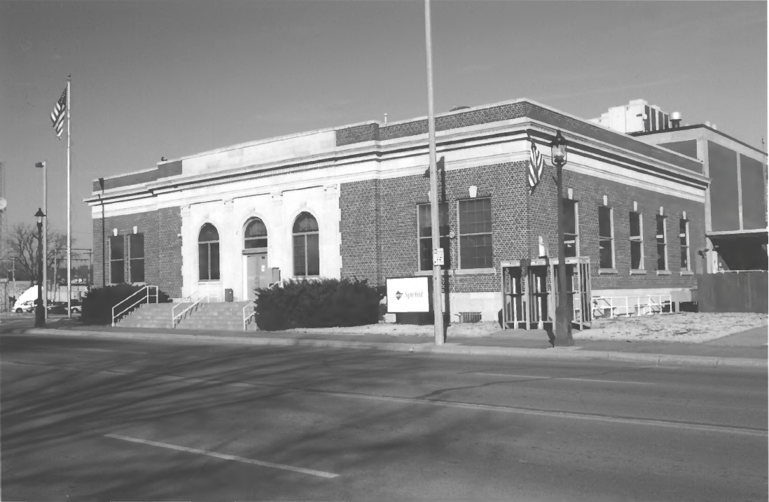
Junction City Downtown District, Geary County, Kansas
