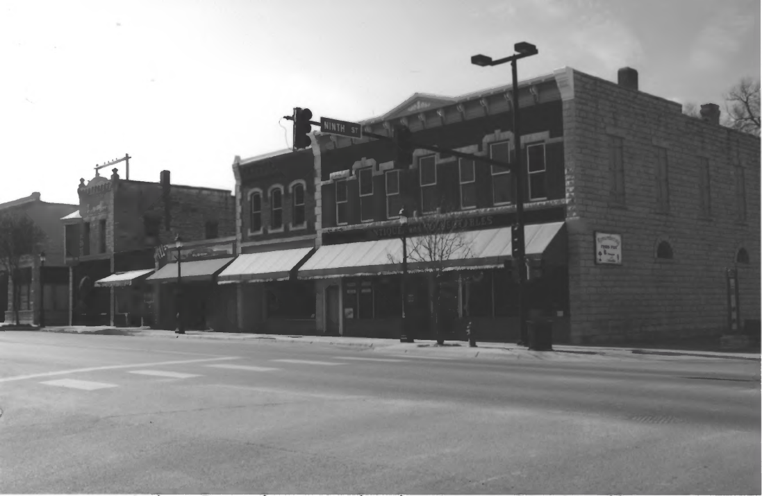
Junction City Downtown District, Geary County, Kansas #11
