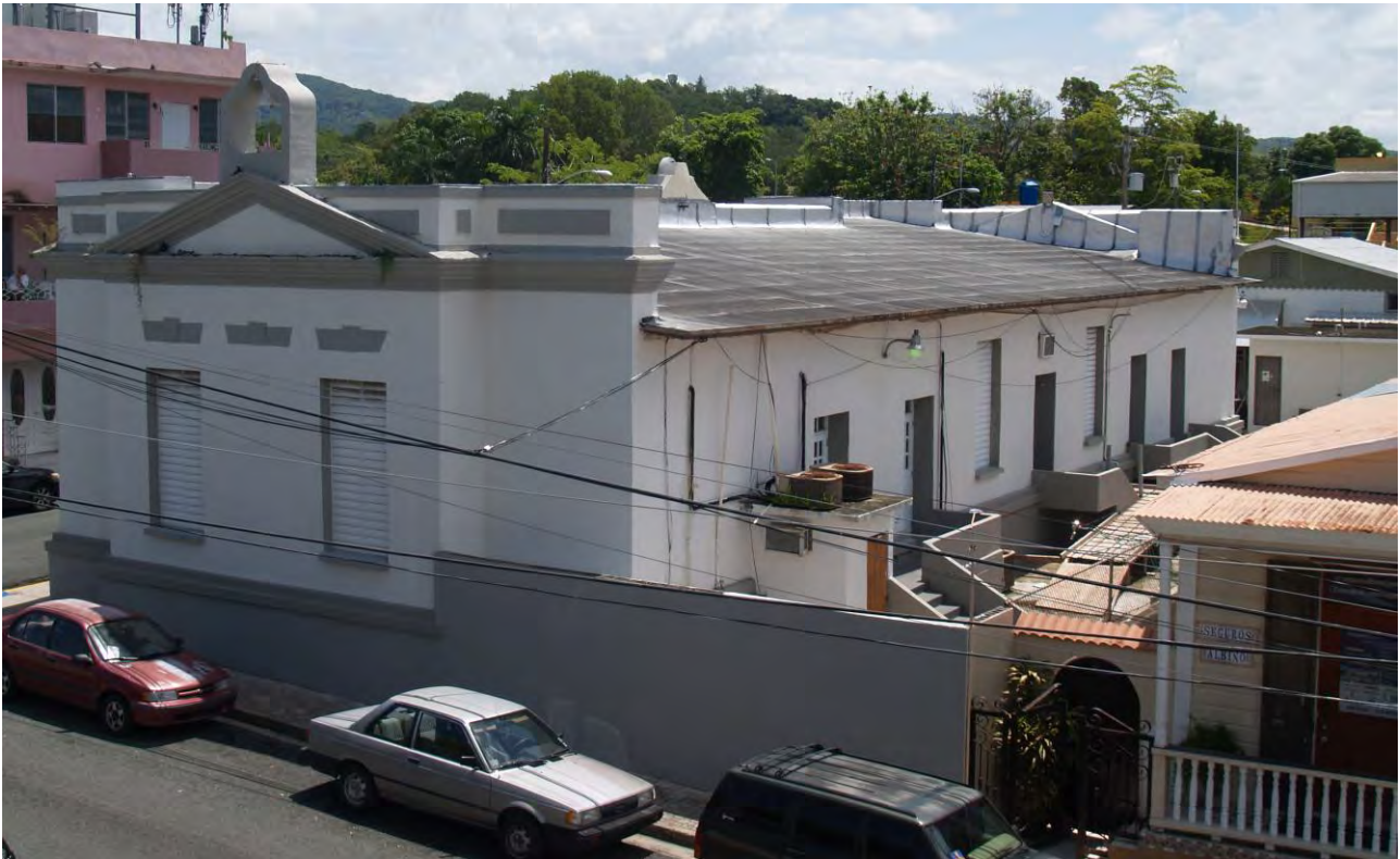
Figure 5. View of the building's roof.
