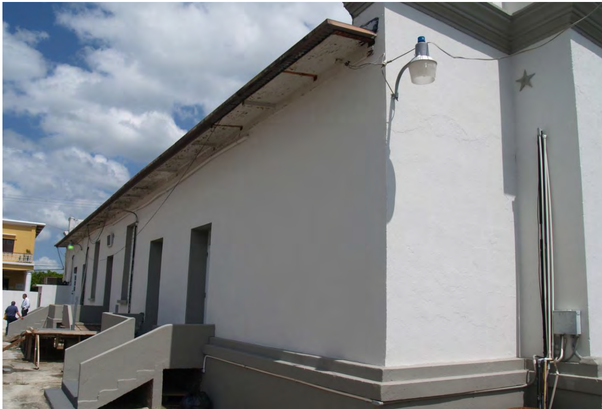
Figure 4. Building's rear (southern façade) showing the concrete stairs and the wooden ramp. The roof wooden panel and corrugated metal is also shown. (Source: Juan Llanes Santos, 2014)
