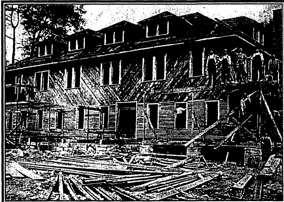
Fig. 4 Shown here under construction, the "Club House" (PI-191) was a center of activity for the management of the coal company.
