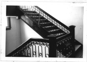
INTERIOR DETAIL - IRON STAIRWAY
