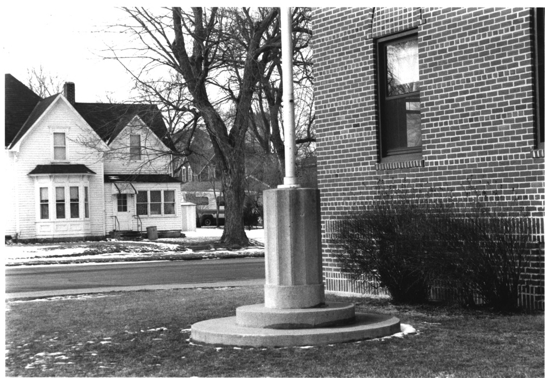
DAWSON ARMORY AND COMMUNITY BUILDING 676 PINE STREET, DAWSON LAC QUI PARLE CO., MN 012459-16
