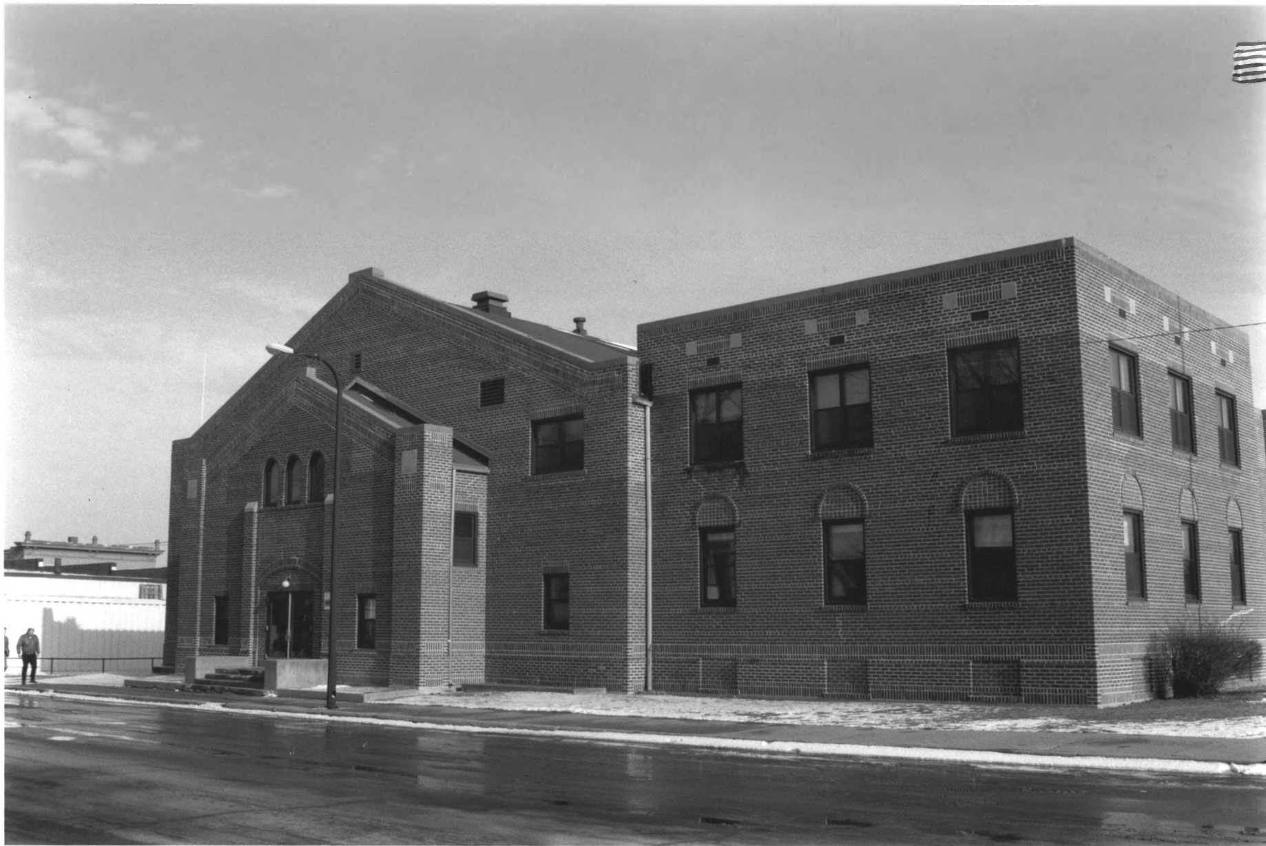
DAWSON ARMORY AND COMMUNITY BUILDING 676 PINE STREET, DAWSON LAC QUI PARLE CO., MN. 012458-8
