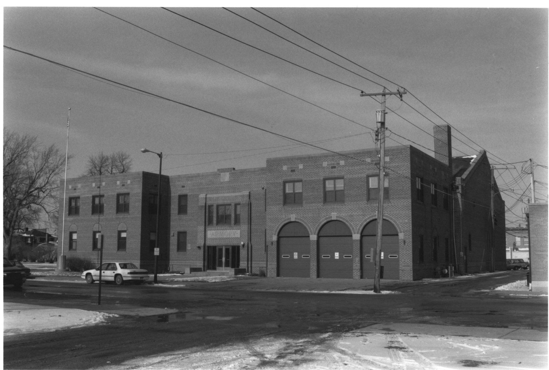
DAWSON ARMORY AND COMMUNITY BUILDING 676 PINE STREET, DAWSON LAC QUI PARLE CO., MN 012458-4
