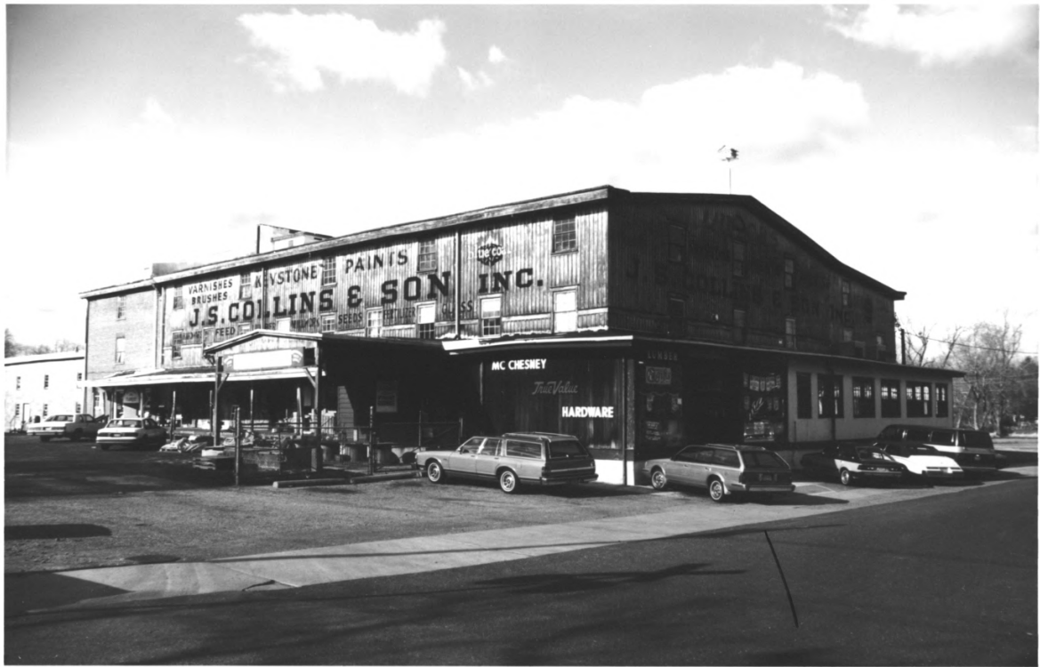
MILL & 3RD STS., MOORESTOWN, BURLINGTON CO., N.J. N-13
