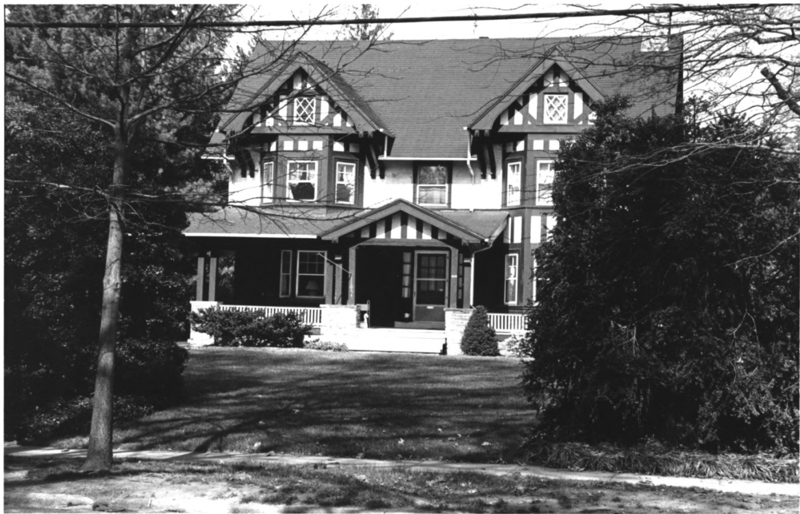
515 CHESTER AVENUE, MOORESTOWN, BURLINGTON CO, NEW JERSEY K-21
