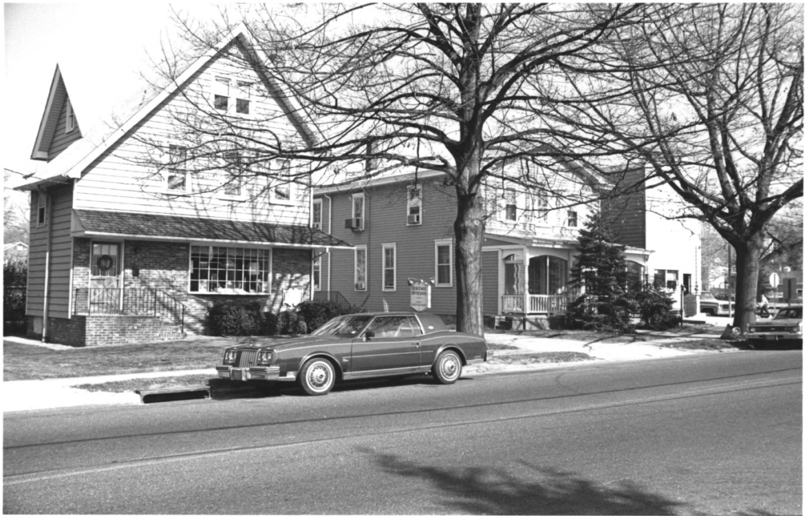
309, 303, 301 CHESTER AVENUE, MOORESTOWN, BURLINGTON CO, NEW JERSEY K-6
