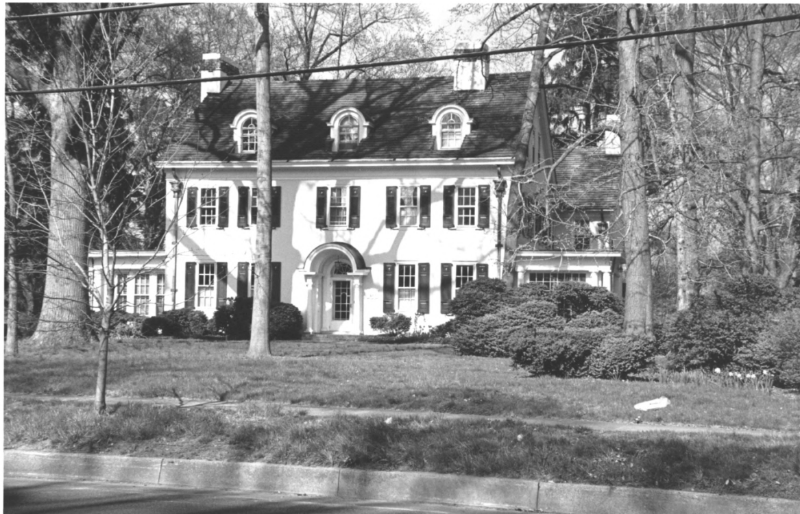
607 CHESTER AVENUE, MOORESTOWN, BURLINGTON CO, NEW JERSEY K-25
