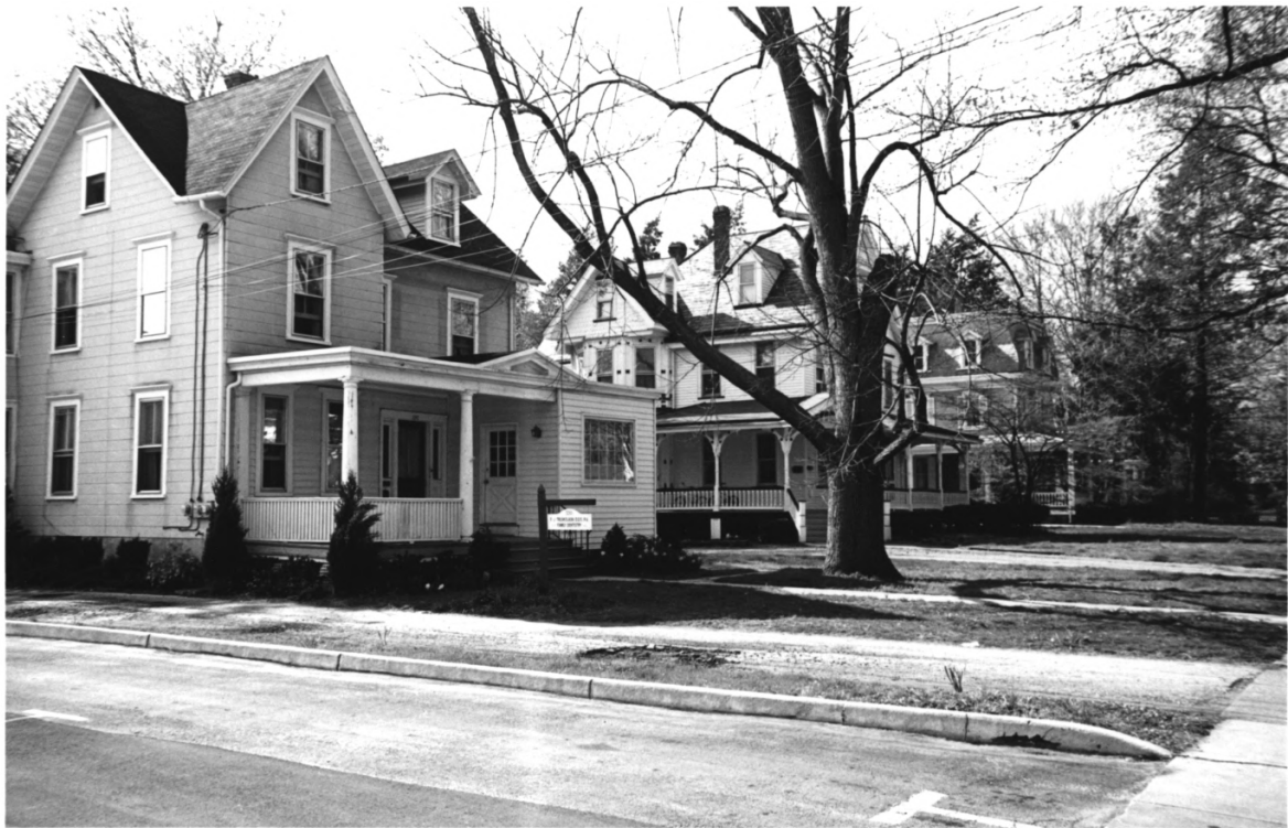
320, 324, 328 CHESTER AVENUE, MOORESTOWN, BURLINGTON CO, NEW JERSEY K-10
