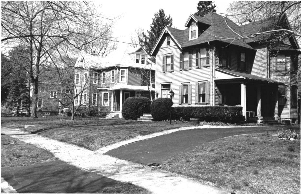
15, 19, 21 EAST OAK AVE. Moo RESTAURANT, BURLINGTON CO, N.J. M-25
