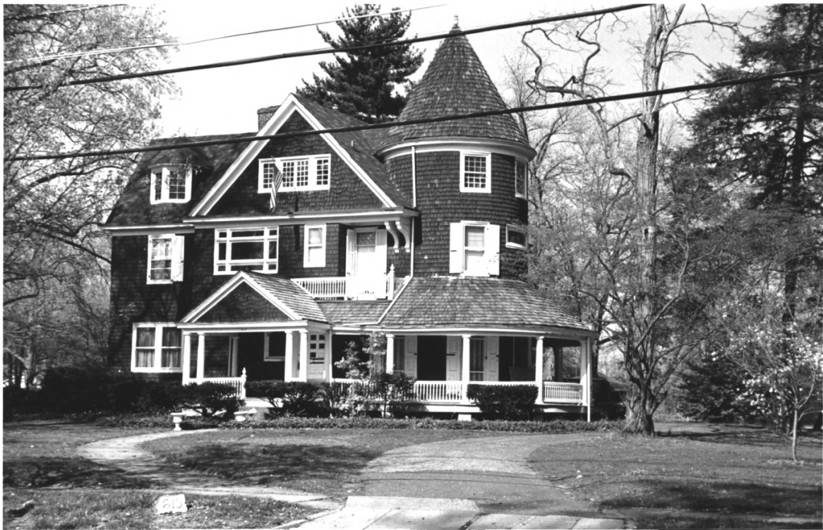
615 CHESTER AVENUE, MOORESTOWN, BURLINGTON CO, NEW JERSEY K-27
