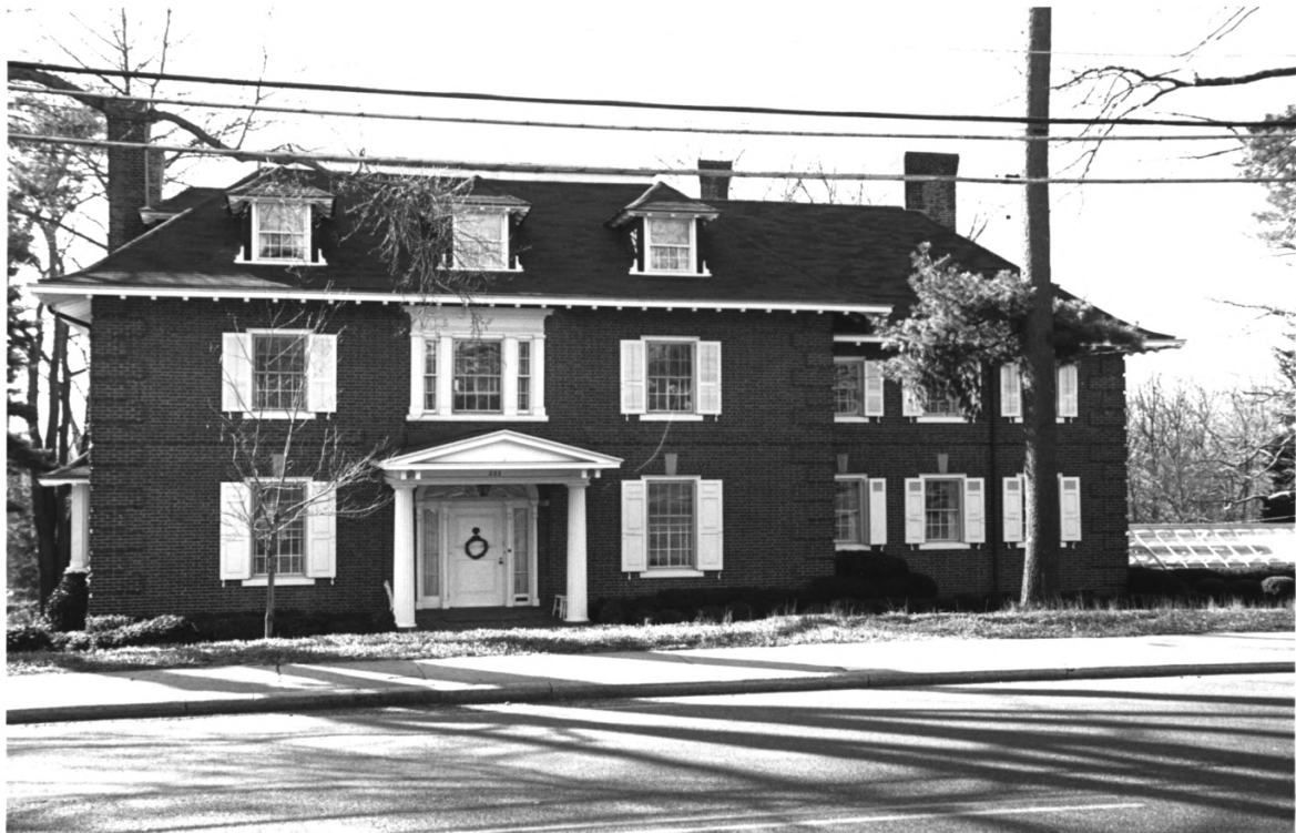
232 E. MAIN ST, MOORESTOWN, BURLINGTON CO., NJ LI LI
