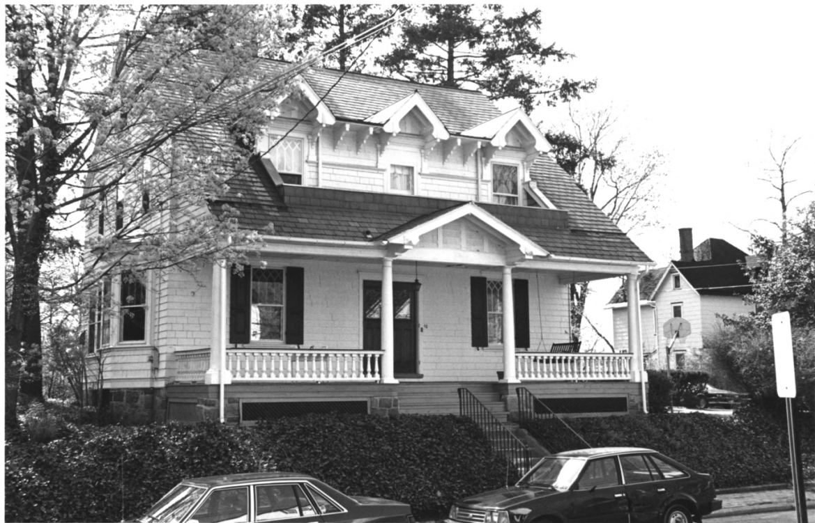
10 HIGH STREET, MOORESTOWN, BURLINGTON CO, NEW JERSEY K-3
