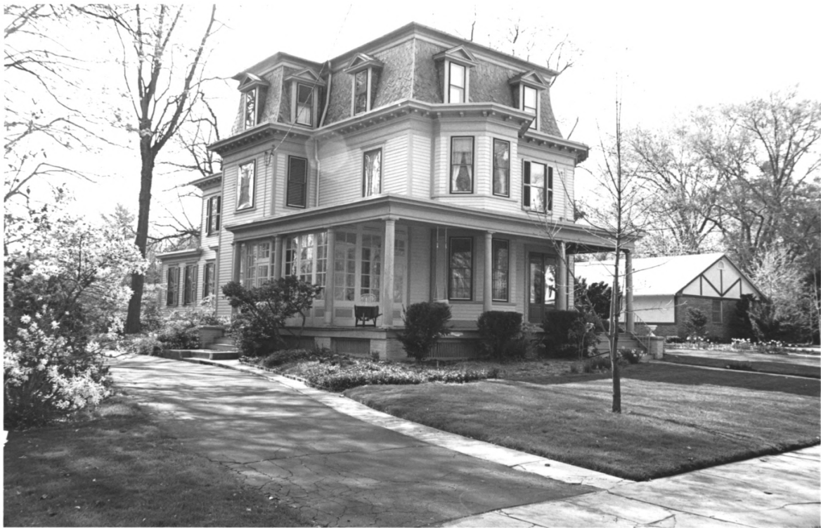
406, 410 CHESTER AVENUE, MOORESTOWN, BURLINGTON CO, NEW JERSEY K-16
