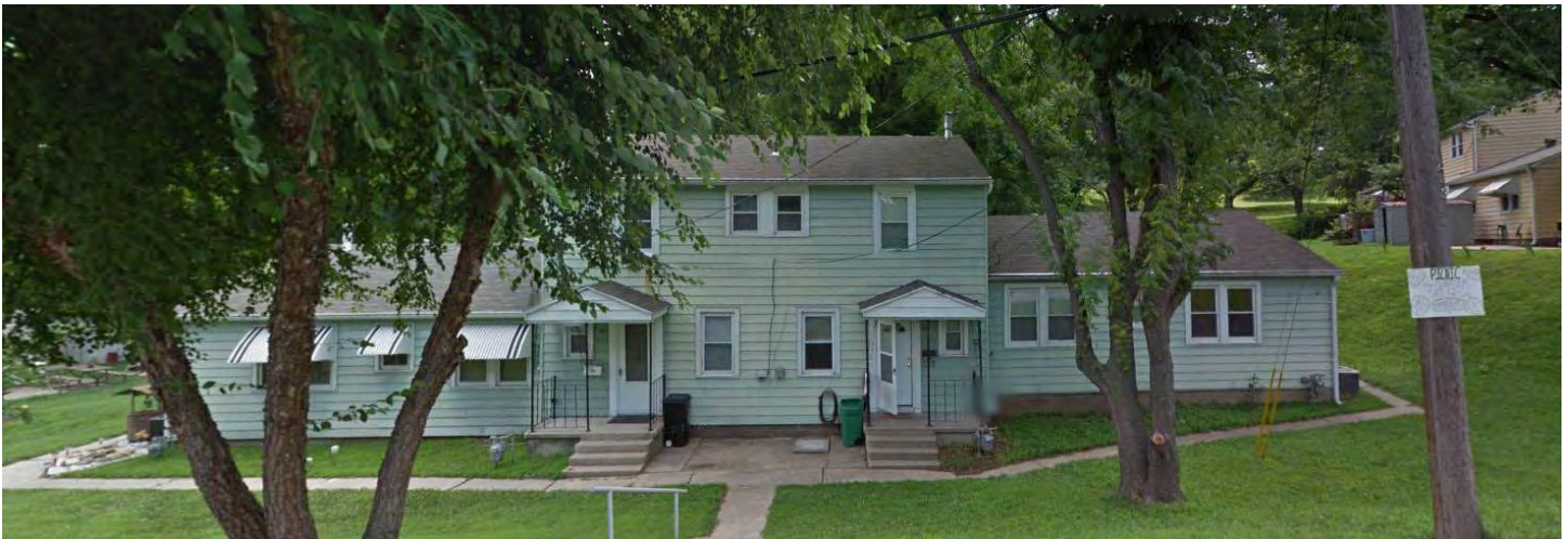
Figure 9. Hovey Place. Typical Building. Google Streetview, 2011.
