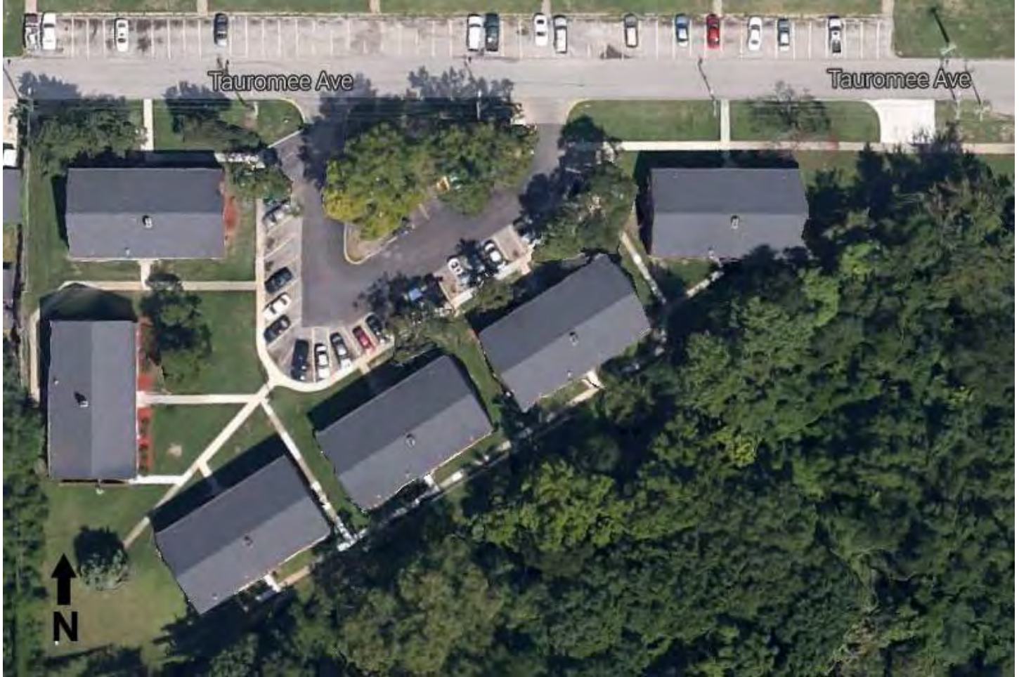
Figure 13. Wyandotte Apartments. Typical Building. Google Streetview, 2011.
