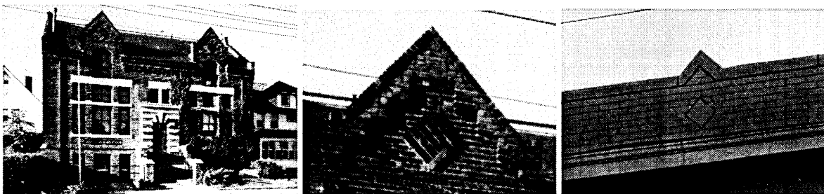
Webster Telephone Exchange building and detail, Broomfield rowhouse detail.
