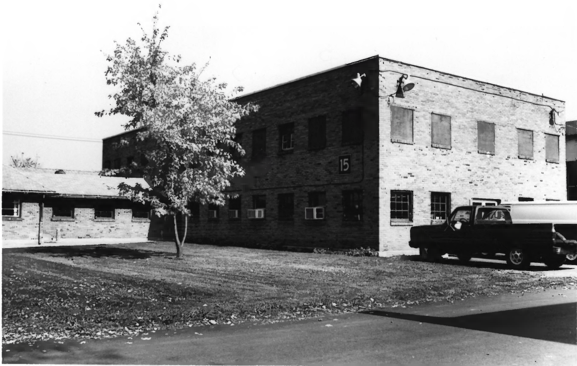
Bldg. #15 Indiana School for the Deaf
