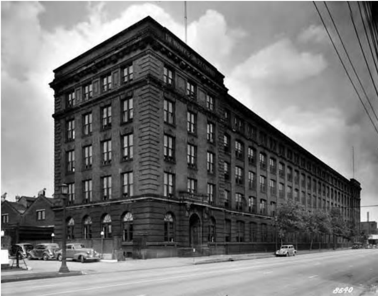
Figure 11. Warner & Swasey Company Building, Photo 1939
