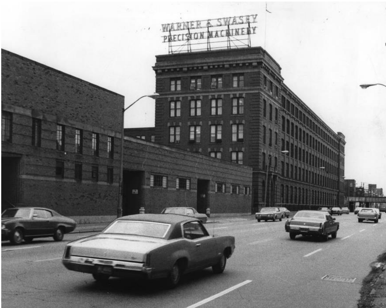
Figure 14. Warner & Swasey Company Building, Photo, 1972
