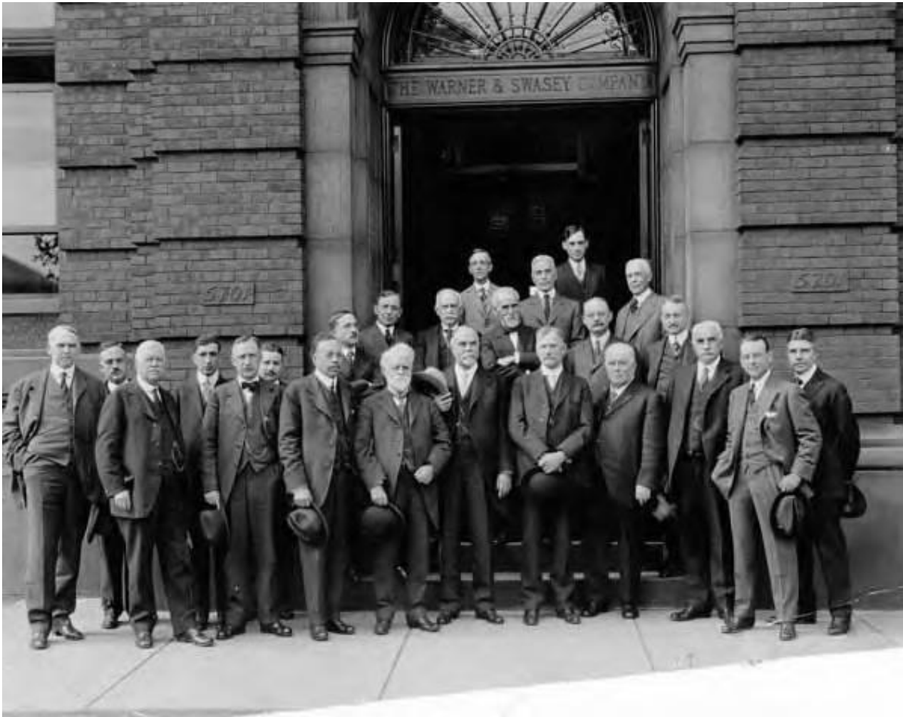
Figure 10. Warner & Swasey Company Building, 5701 Carnegie Ave., Building Entry, Photo 1916
