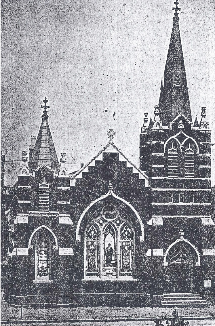
Figure 7: St. Paul's Church after its 1902 renovation. Source: St. Clair County Centennial Edition (1914).
