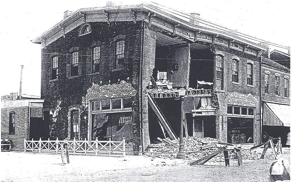
Figure 14: The Oliver C. Joseph Chrysler Dodge building at 219-23 W. Main Street after a streetcar struck the building in 1923. Source: Belleville Historical Society.
