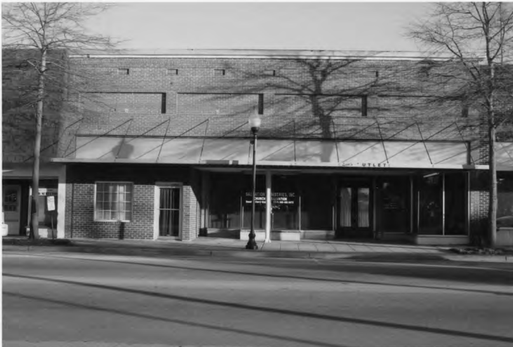
22. Manning Commercial Historic District 13 West Boyce Street, Manning Clarendon County, South Carolina
