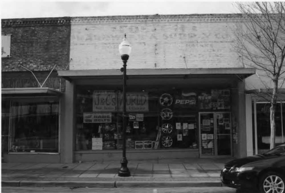
56. Manning Commercial Historic District 31 North Brooks Street, Manning Clarendon County, South Carolina
