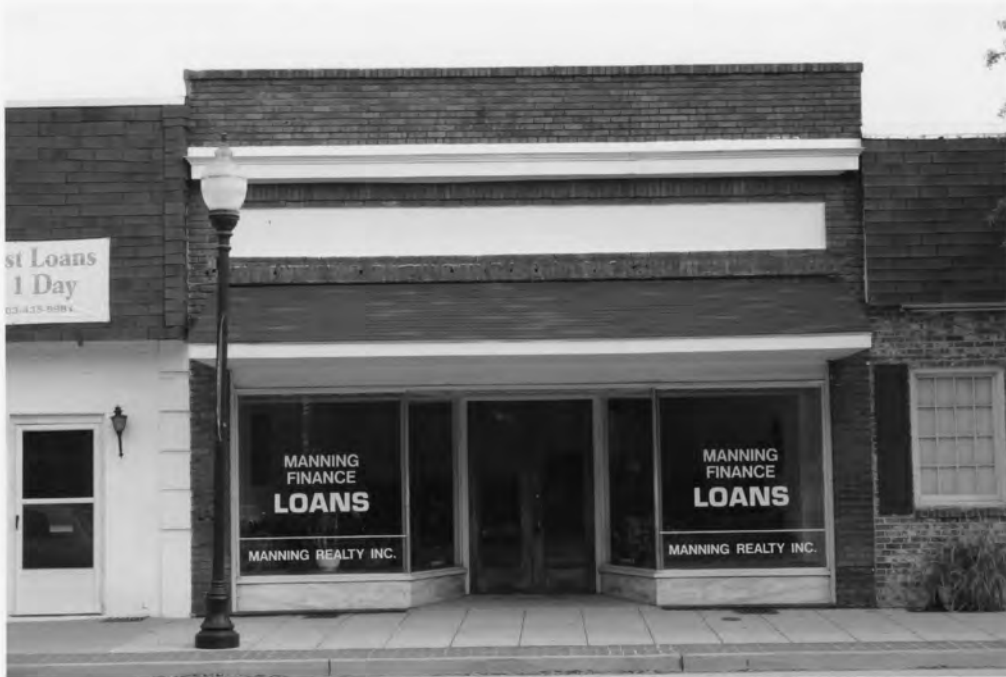
21. Manning Commercial Historic District 21 West Boyce Street, Manning Clarendon County, South Carolina
