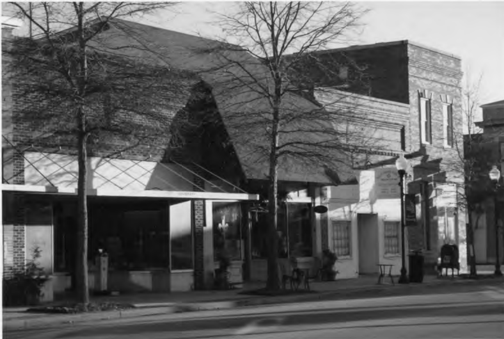
23. Manning Commercial Historic District 7, 5, 3 and 1 West Boyce Street, Manning Clarendon County, South Carolina
