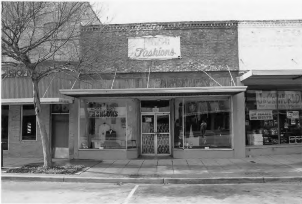
57. Manning Commercial Historic District 27 North Brooks Street, Manning Clarendon County, South Carolina
