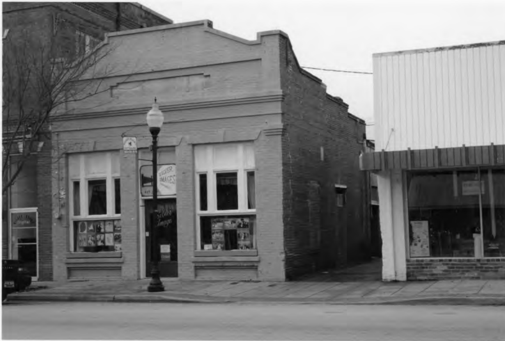
61. Manning Commercial Historic District 9 North Brooks Street, Manning Clarendon County, South Carolina
