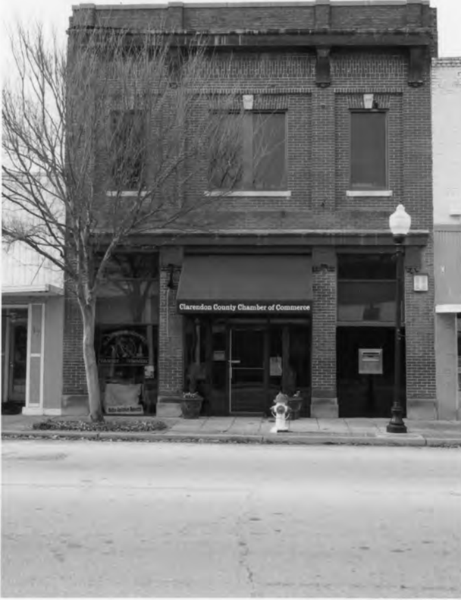
60. Manning Commercial Historic District 19 North Brooks Street, Manning Clarendon County, South Carolina
