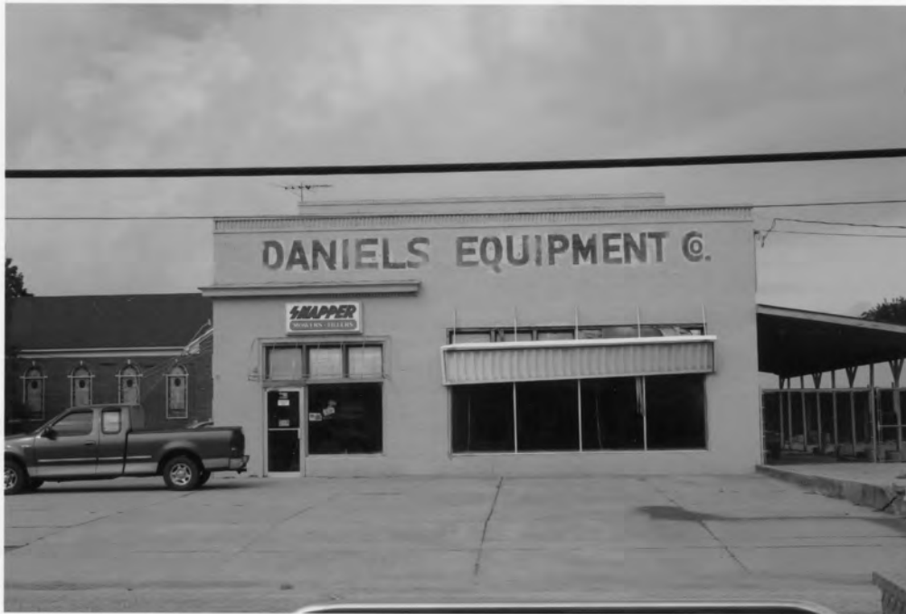
12. Manning Commercial Historic District 17 North Mill Street, Manning Clarendon County, South Carolina
