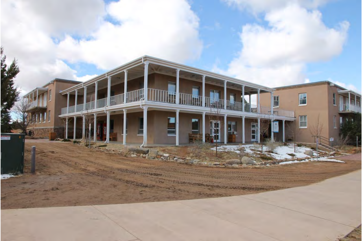
32 of 35. Lower Dormitories, photographer facing southwest
