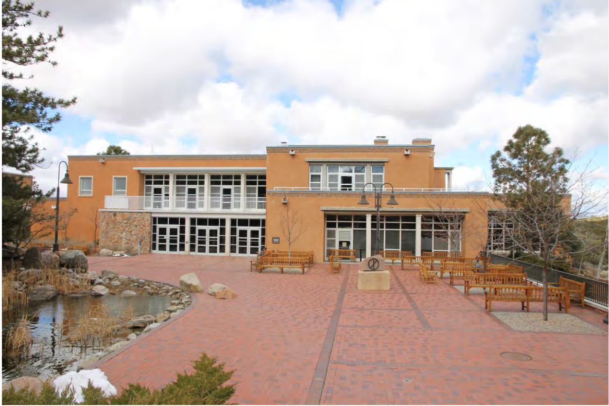
5 of 35. Peterson Student Center, photographer facing west
