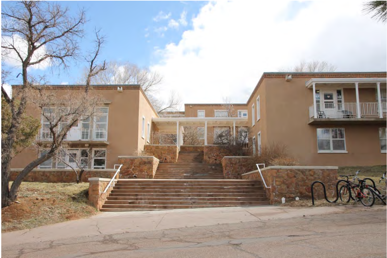
26 of 35. Upper Dormitories, west facades, photographer facing east
