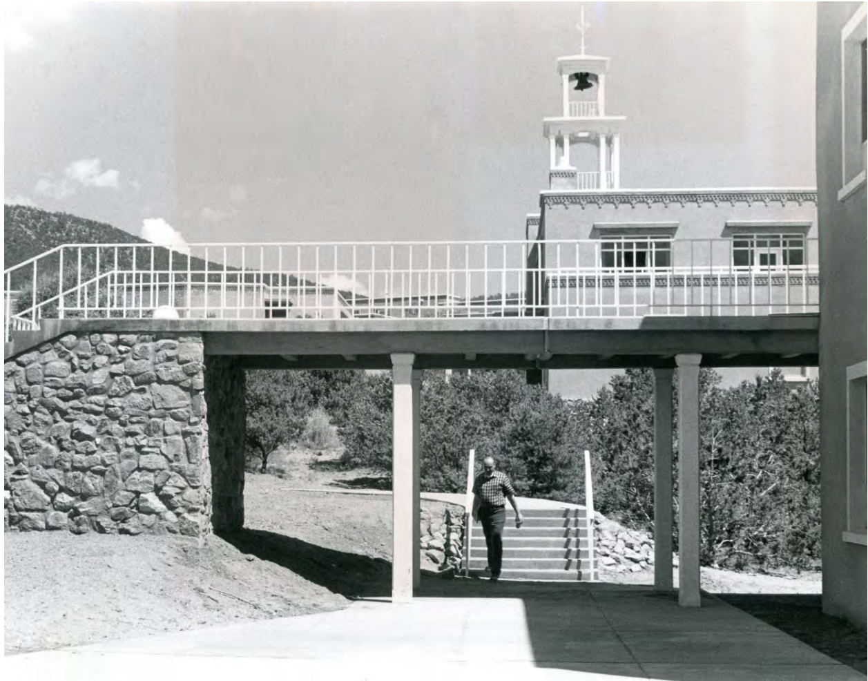
Figure 6. St. John's College in 1964, with second-floor walkway (not extant) from Fine Arts Building (far right) to Peterson Student Center (not seen), and Weigle Hall (center right)
