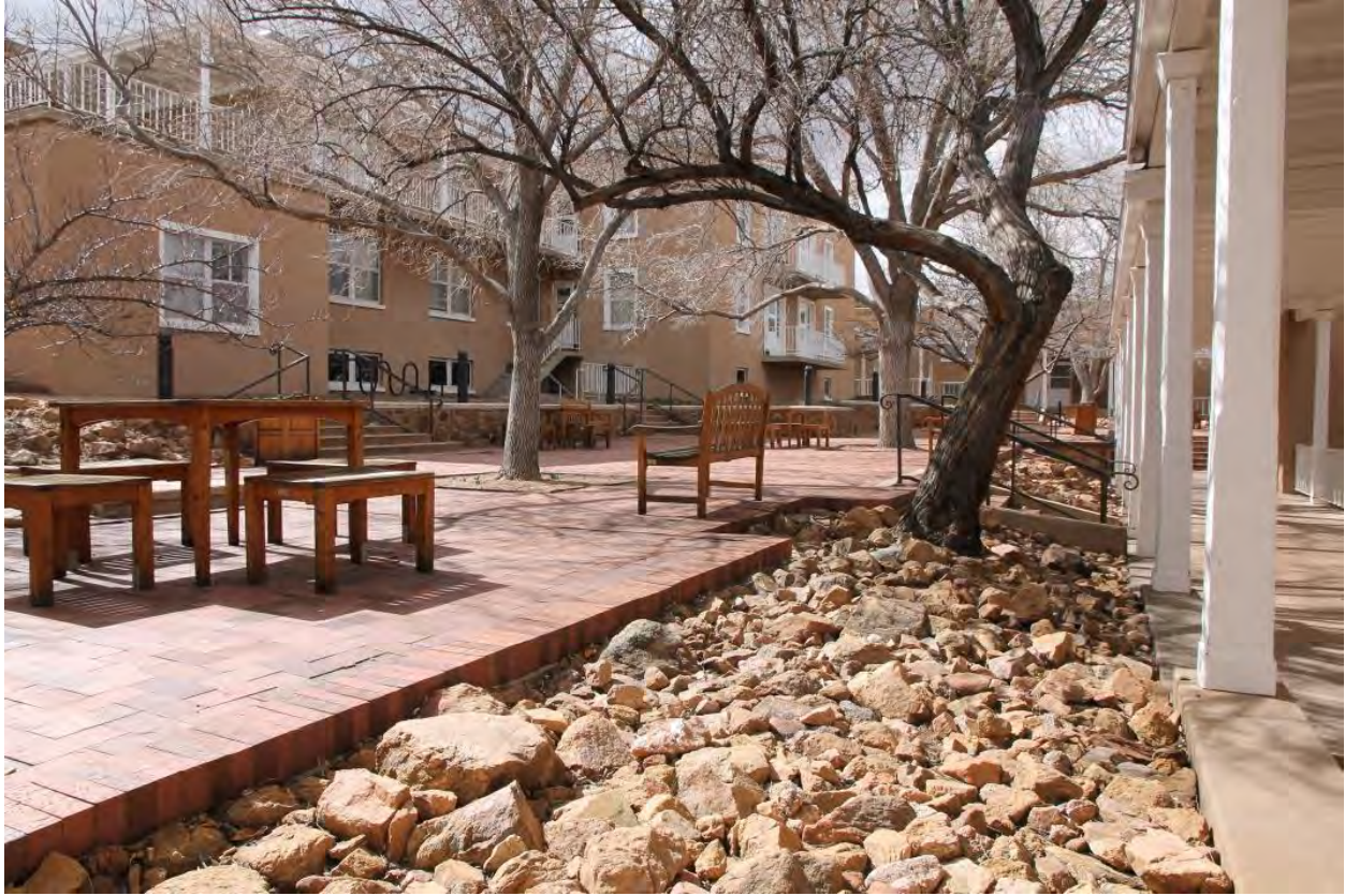
28 of 35. Upper Dormitories, north placita, photographer facing south
