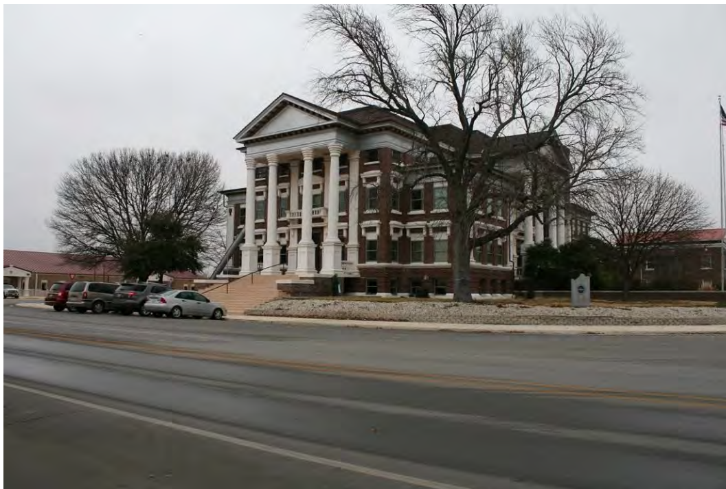
Photo 5: Looking northeast at west and south elevations of courthouse and west elevation of jail
