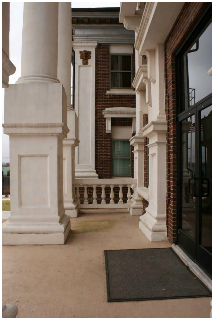
Photo 6: Looking east at details of north porch
