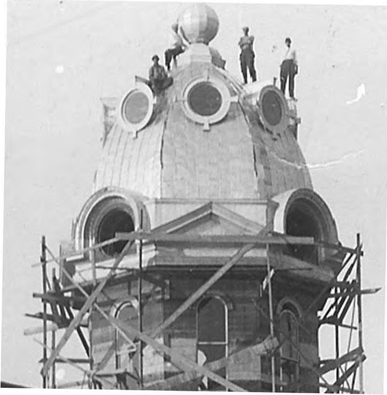
Figure 5: Cupola under construction, 1913. Courtesy Montague County Historical Commission.
