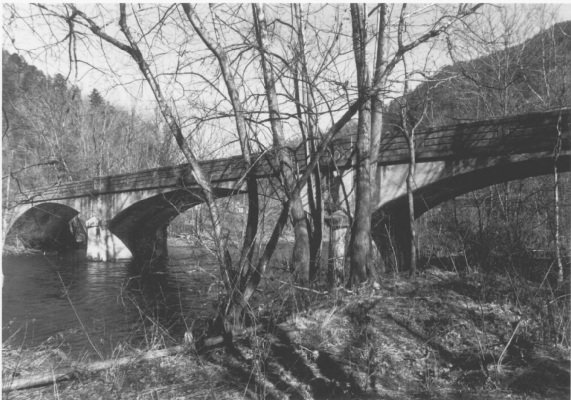
Walland Bridge, Blount Co., TN, Photo 1 of 2
