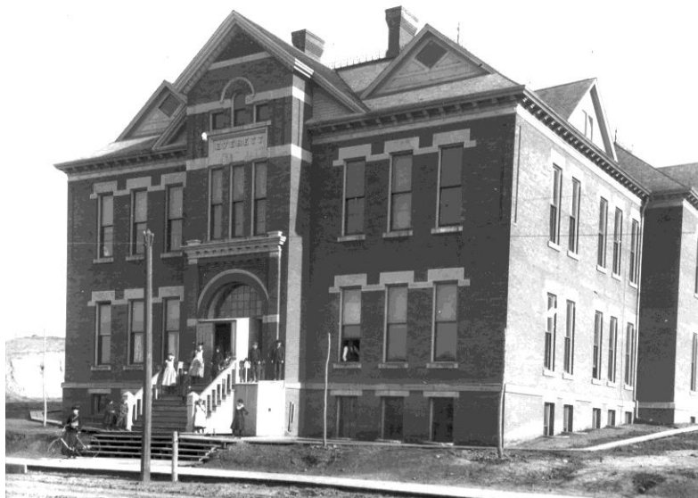
Figure 2: Everett School showing the original 1888 building and 1891 addition (Sioux City Public Museum, date unknown).
