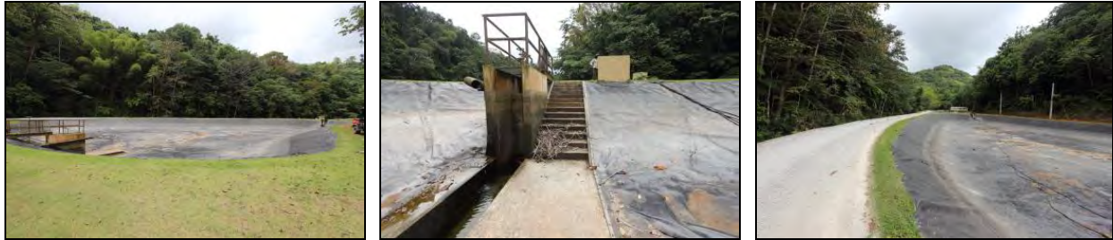
Picture 27, 28 and 29. Views of the grow-out pond #4 (CC4) emptied for routine maintenance. The photos were taken from the interior service road, close up of its fish kettle and from the exterior service road (close to the river bed).
