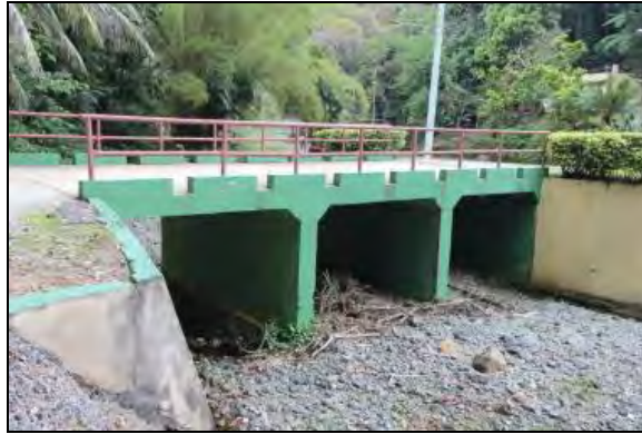
Picture 40. Three span concrete bridge over the Maricao River.
