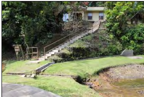
Pictures 33. Concrete stairway and spawning pool CR3 with Administration building in the foreground a top of the hill.
