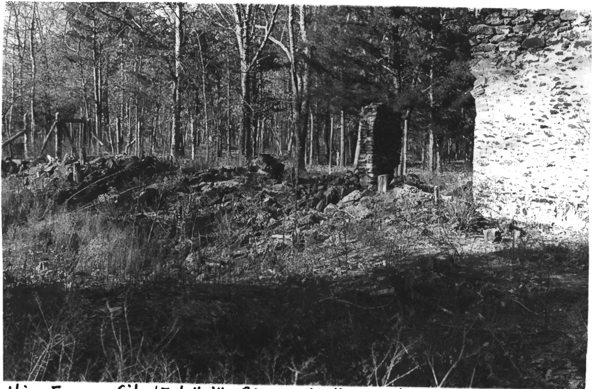
2. Melting Furnace Site/Estellville Glassworks H.D., Estell Manor City, Atlantic County, New Jersey
